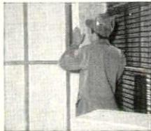
Gimco Sealal Bats fit standard spaced studdings in buildings under construction.
