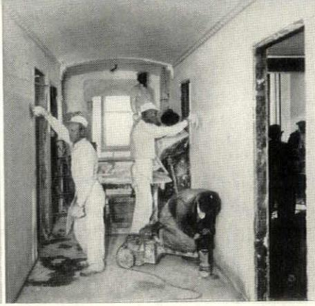
... the ductwork was "furred in", a new ceiling built ...
