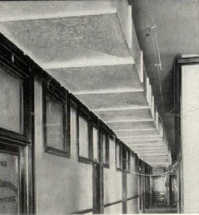
... ductwork was suspended to carry the conditioned air ...
