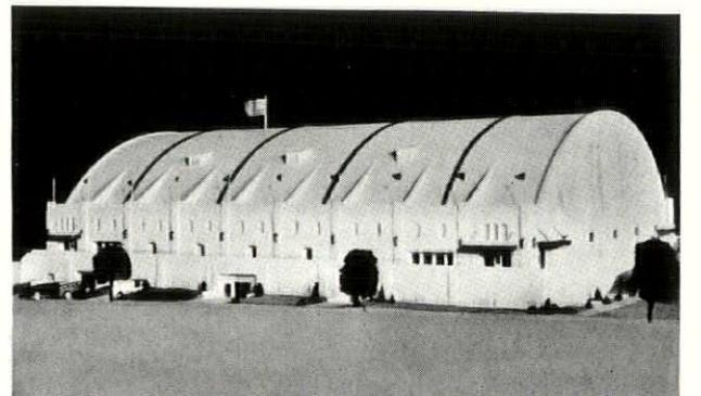
Exterior of the Hershey Sports Arena. Heating pipes are located behind alternate rows of seats. Ventilating fans change air every 15 minutes.
