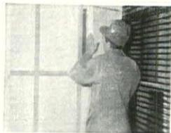
Gimco Rock Wool Sealal Bats fit standard spaced studdings in buildings under construction.
