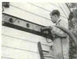
Gimco Rock Wool is quickly blown into empty wall and ceiling spaces in present homes.
