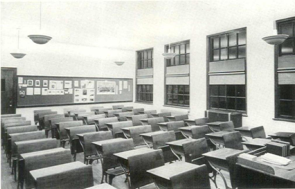
Figure 6. A typical classroom equipped with six 500-watt Mazda lamps in totally-indirect luminaires. Under average service conditions an illumination of the order of 20 footcandles will be received on the desks throughout the room.
