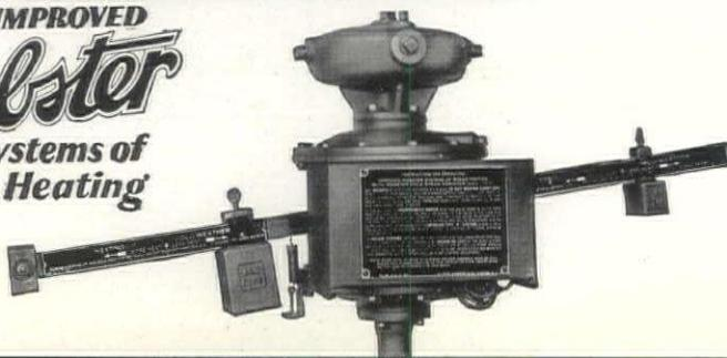
The Webster Hylo Steam Variator—a simple, rugged central control—regulates the heating of 11 New York State school buildings on this page. The Hylo Steam Variator (illustrated) automatically throttles a rugged motor-operated valve in the steam main.
