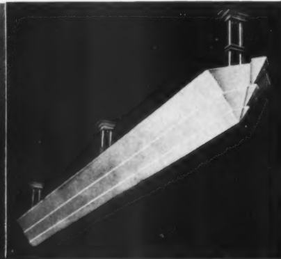
Above— Indirect troughs in auditorium, University of Maryland Hospital, Baltimore, Md. Smith and May, Architects
