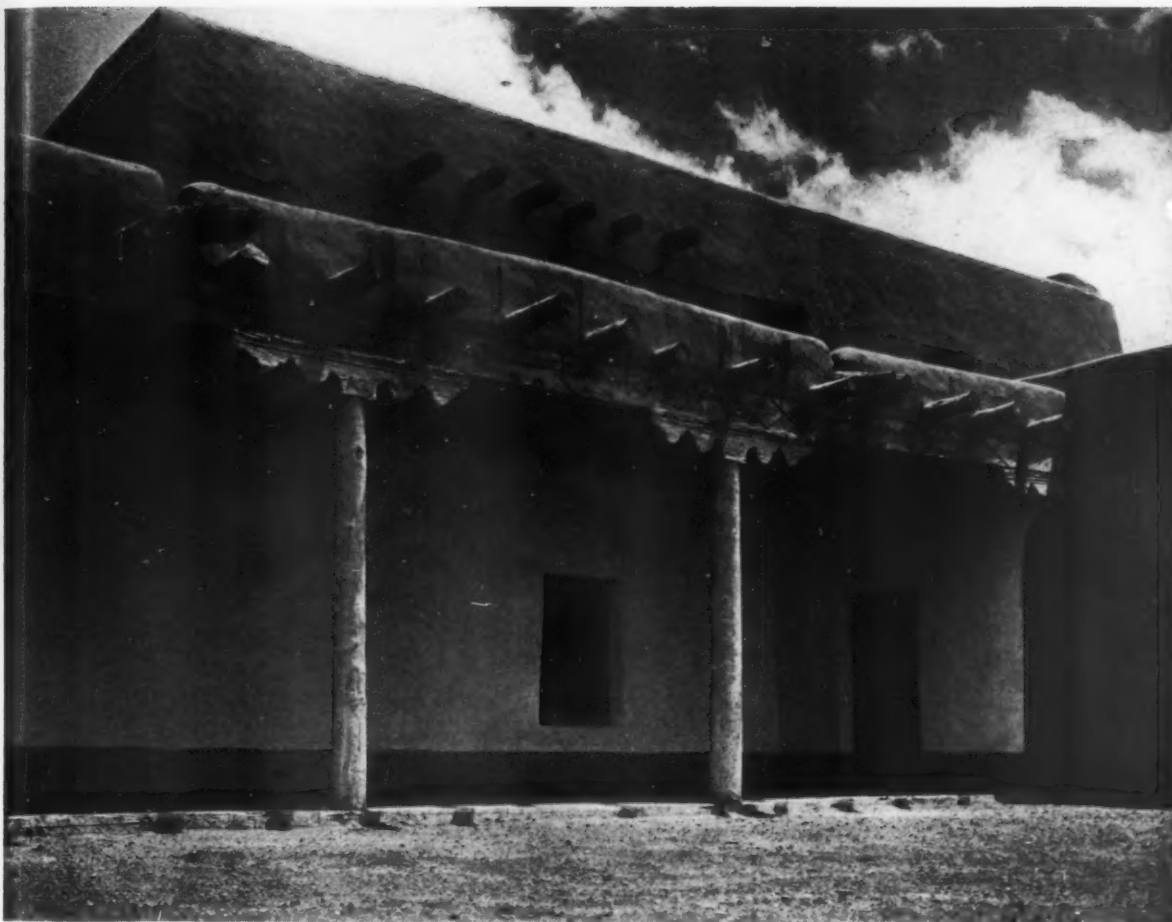
Detail of entrance porch, house of Miss Amelia B. Hollenback, Santa Fe, New Mexico. John Gaw Meem, architect. On facing page: plan and general view of the same house. Most of the exterior walls are adobe, some of them over two and one-half feet thick
