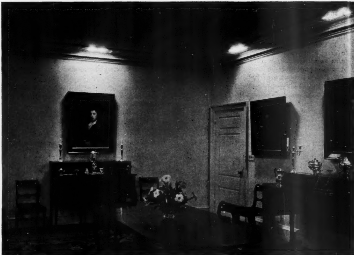
Prismatic lenses in ceiling light boxes used for side-wall lighting in apartment of H. H. Porter; Rosario Candela, Architect. Note that unit placed over door for symmetrical spacing projects light to the right as well as toward wall
