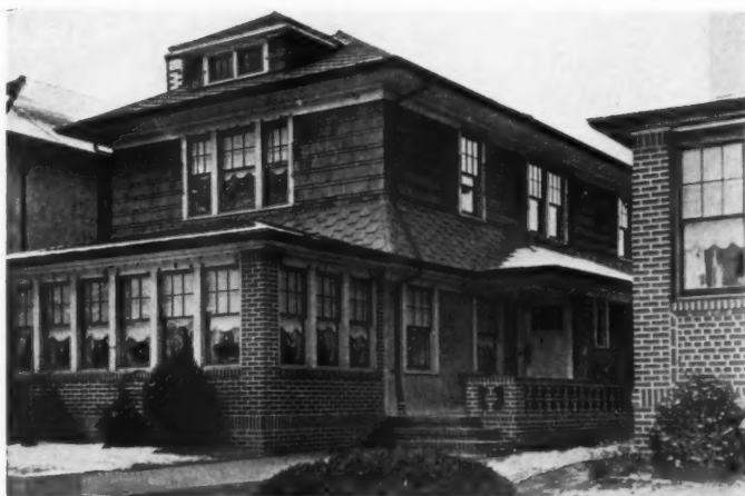
Mr. Max Troy's home, Brooklyn, N. Y., in which he installed a Model R, vertical rotary type, domestic Petro-&-Nokol oil burner
