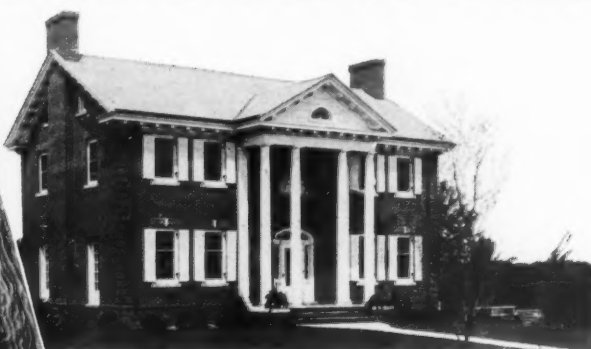
Home of Dr. J. J. Noonan, Marshalltown, Ia. Architect, R. J. Prescott. Roofed with 2,000 square feet Jade Green Eternit Gothics.
