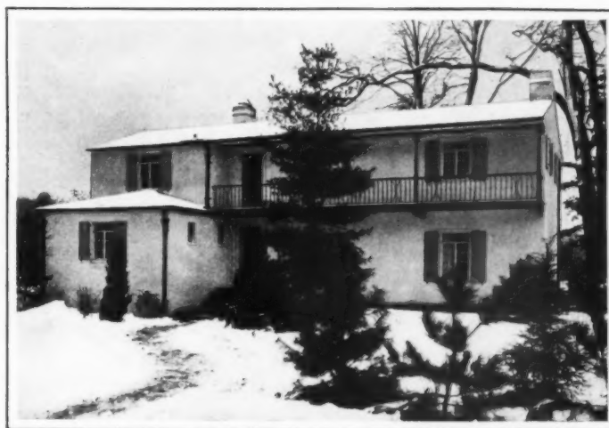
The prize-winning Model Home, at Sleepy Hollow Manor, Tarrytown, N. Y. Built by Sleepy Hollow Manor, Inc. Architect, H. Roy Kelly.
