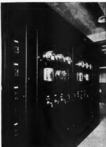
A Westinghouse Nofuze-equip'ed switchboard in Fitzgerald-Mercy Hospital, Darby, Pa., provides permanent protection of the building's circuits, varying from 30 to 600 amps. capacity. It requires only approximately 2 1/2 the space of the conventional type switchboard. Architect—Hoffman-Henon Co., Philadelphia.
