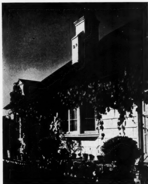
Residence at Los Angeles, California. Leland F. Fuller, A.I.A., Architect and Owner. Cabot's Old Virginia White on side walls, DOUBLE-WHITE on exterior brick, Cabot's Creosote Shingle and Wood Stains (Dark Blue) on roof.
