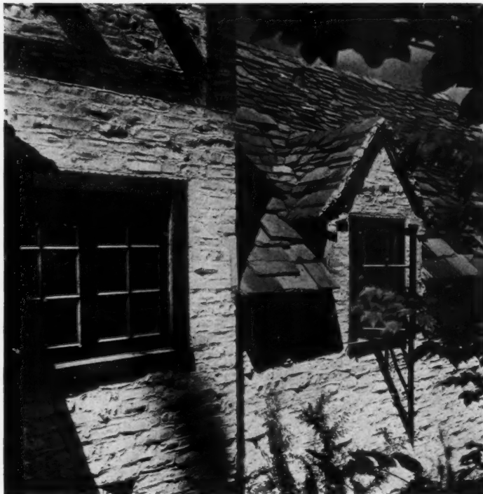
Detail of Dormer in Garage Wing, Showing Texture of Roof and Half-Timbering
