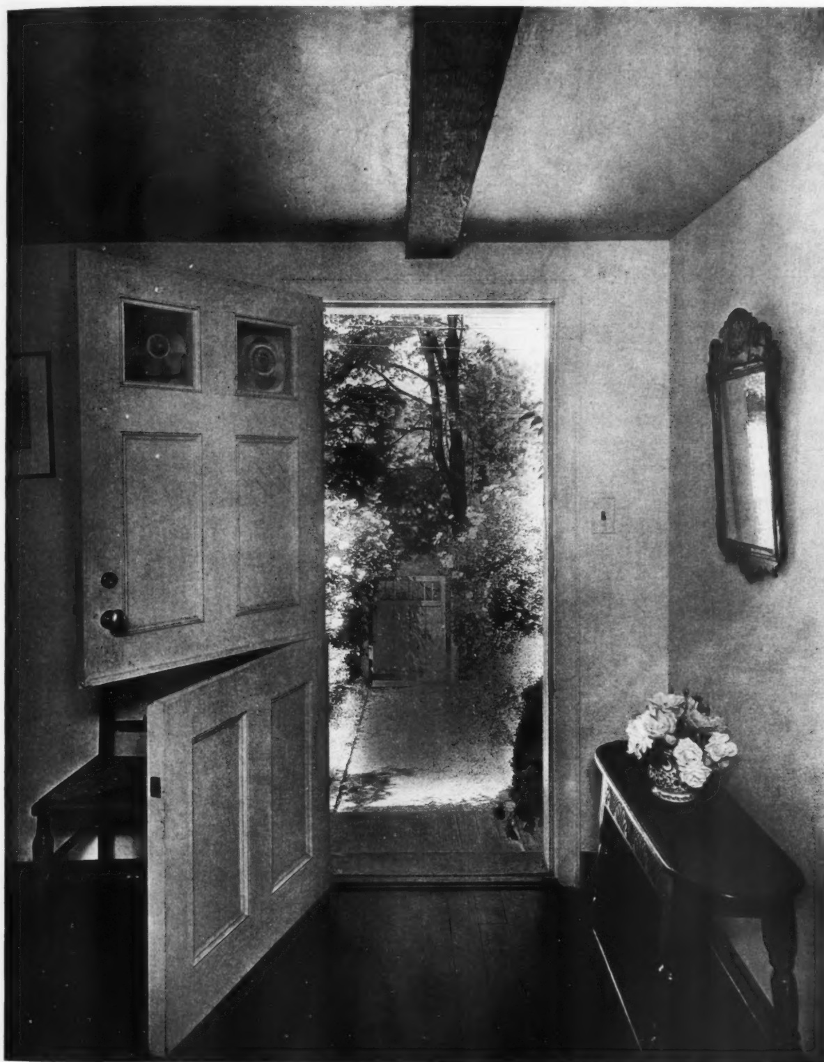
The diminutive scale of the interior is even more emphatic than that of the exterior. Many of the door openings were and still are only five feet ten inches in height. The entrance door is six feet high. Note the unusually low ceiling height of the first story as shown above
