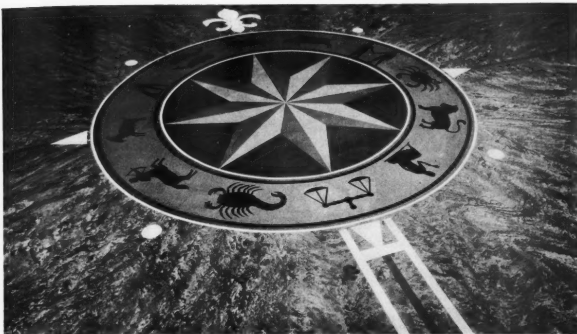
This inlaid compass point of special design is in the Topeka High School, Topeka, Kansas, Jameson W. Williamson & Co., architects. The field is of marbled linoleum laid in segments so that the striations point to the center. Colors used are: 1. Light yellow 2. Light tan 3. Terra cotta red 4. Light blue 5. Chocolate brown 6. Light brown 7. Marbled in gray-brown tones
