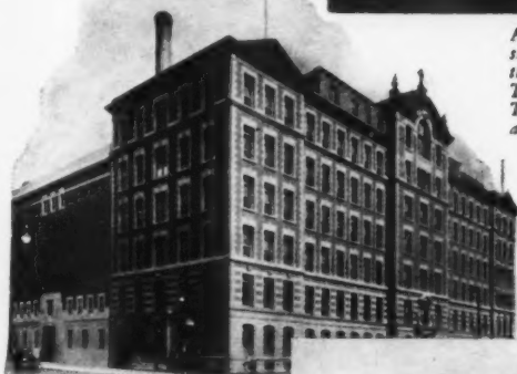
St. Vincent's Hospital, 11th St. & 7th Ave., New York, N. Y. Three 350 H.P. Babcock & Wilcox Boilers fired by 9 Todd mechanical natural draft type burners.
