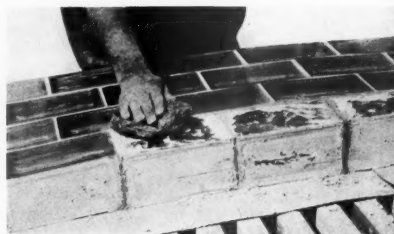
At right: Mortar is applied to the Owens-Illinois glass block the same as in the case of clay bricks. . . Lower left: Joints are tooled to seal their surface and increase water tightness. . . Lower right: The surface of the blocks is cleaned with steel wool after erection
