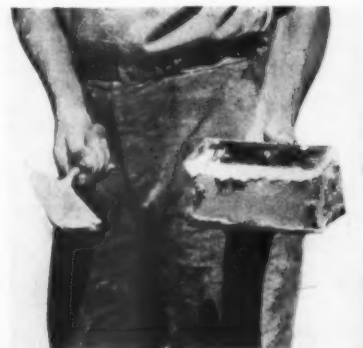
At right: Mortar is applied to the Owens-Illinois glass block the same as in the case of clay bricks. . . Lower left: Joints are tooled to seal their surface and increase water tightness. . . Lower right: The surface of the blocks is cleaned with steel wool after erection
