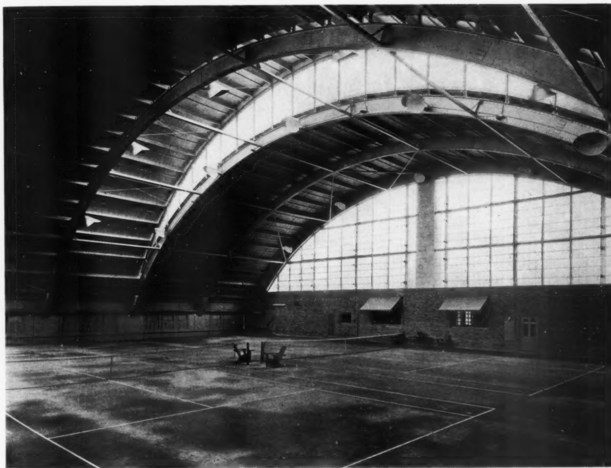
The Roof is Arched Longitudinally to Provide Maximum Height Over the Nets
