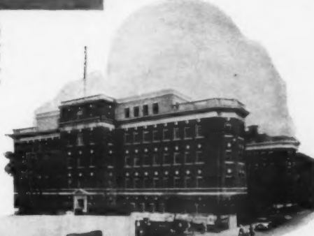
Harlem Hospital, 136th St. & Lenox Ave., New York, N. Y. Four 340 H.P. Water Tube Boilers fired by 12 Todd mechanical natural draft type burners.
