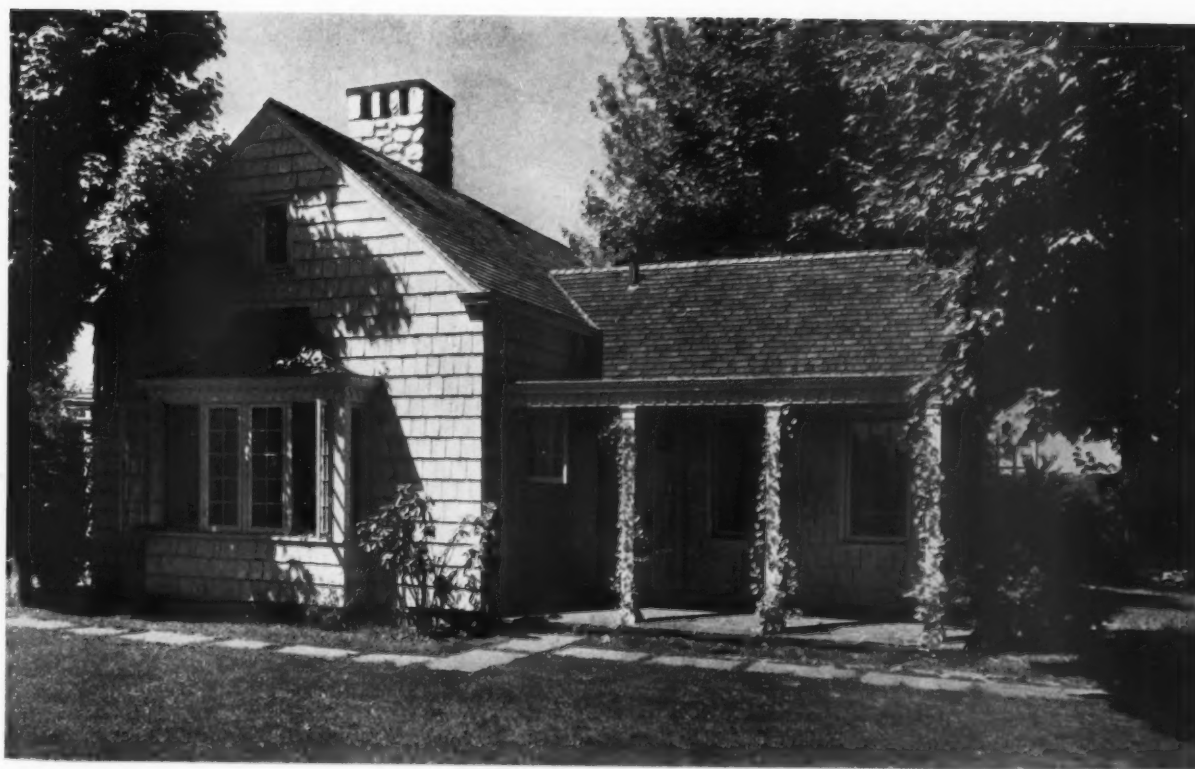
The gardener's cottage stands by the main entrance gate. The field stone wing contains the gardener's office shown on the plans of the following page
