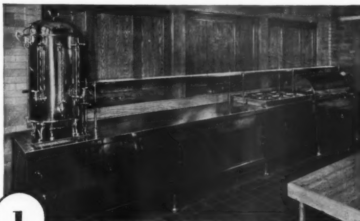
Monel Metal food service equipment in faculty cafeteria room of the Benjamin Franklin Junior and Senior High School, Rochester, N. Y. This combination counter, steam table, warmers and coffee urn was installed by Holderle Bros., Inc., Rochester, N. Y. Gordon & Kaelber, Architects.
