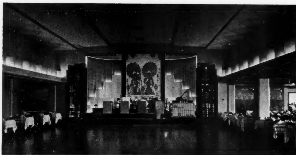
THE CEILING has no painted decoration, the patterns being a lighting effect secured by incorporating metallic cutouts in the indirect illuminating fixture. Julliard School of Music; A. L. Harmon, architect
