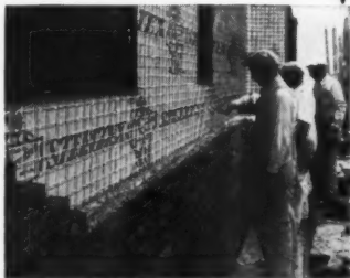
Bricks are laid one inch away from STEELTEX 38-16. This one-inch space is filled in with bricklayer's cement-mortar,—the galvanized, copper-bearing wire reinforcing mesh of STEELTEX becomes embedded in this back-up slab.
