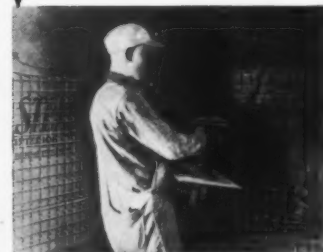
Ribbed STEELTEX Lath holds the wet plaster with instant bonding action. Plaster flows under and around the galvanized, copper-bearing wire reinforcing mesh which becomes completely embedded,—giving lifetime walls and ceilings.
