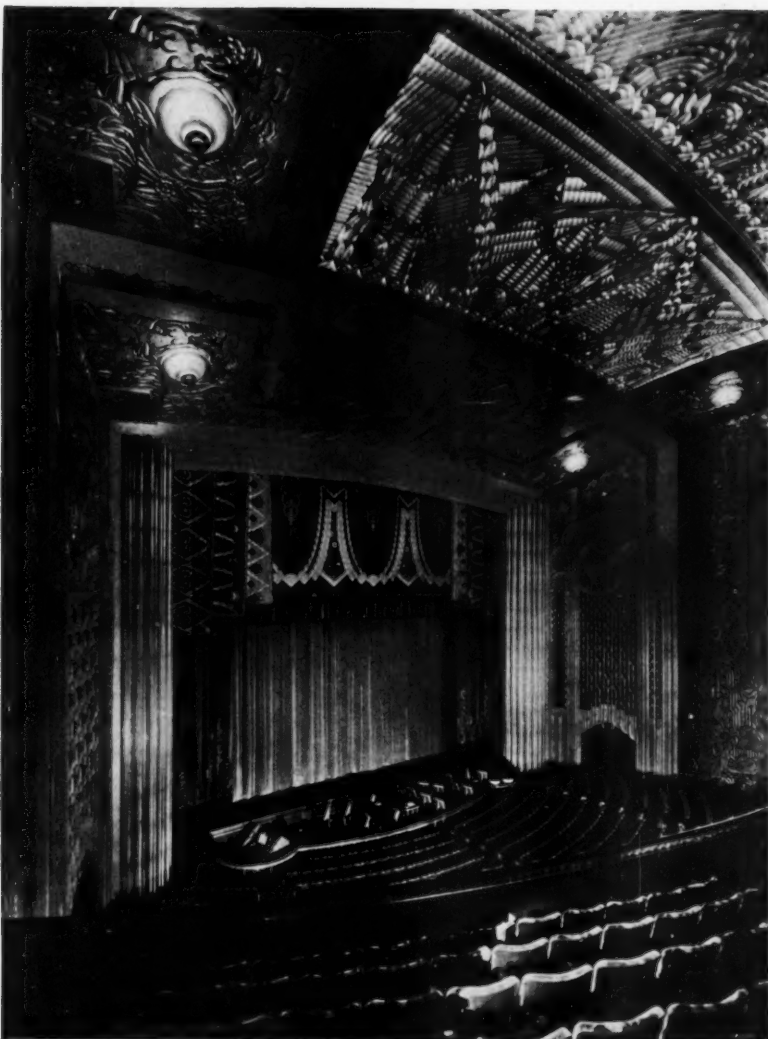
PROSCENIUM of the Paramount Theatre, Oakland, Cal. It is composed of bent sheet metal strips which are lighted from behind. A detail of the proscenium is shown at the right. J. R. Miller and T. L. Pflueger, architects
