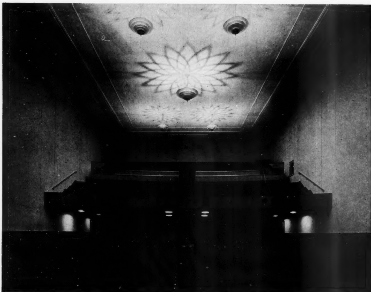
THE CEILING has no painted decoration, the patterns being a lighting effect secured by incorporating metallic cutouts in the indirect illuminating fixture. Julliard School of Music; A. L. Harmon, architect
