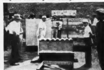
(Below) STEELTEX and one inch cement applied direct to studs is twice as strong as diagonal sheathing and siding.
