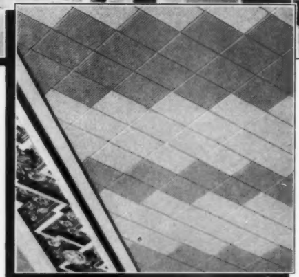
● Detail of the Acousti-Celotex ceiling of the Santa Monica Branch, Bank of America, Santa Monica, Calif. — Architects, Kumpel & Erkes.
