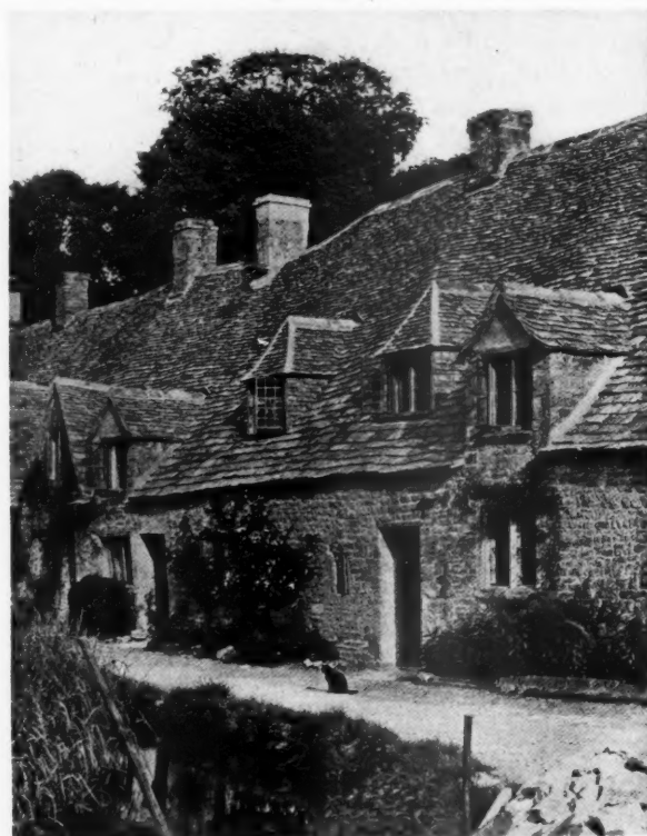
Arlington Row, Bibury, Gloucestershire. From "Small Stone Houses of the Cotswold District"
