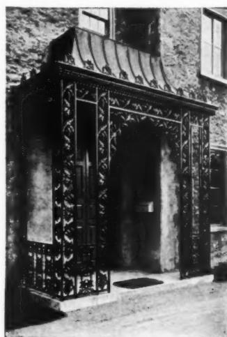
The same entry, after Smyser-Royer cast iron veranda was installed.
