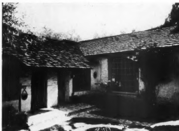
Adobe House, Pasadena, California. Roof of \frac{3}{4} " to 1" x 25" Hand Split Red Cedar tapered shakes machine-dipped in three shades (brown) of Cabot's Creosote Shingle and Wood Stains.
