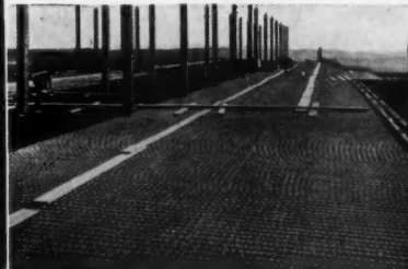
STEELTEX Floor Lath is unrolled over the joists. The illustration above shows STEELTEX Floor Lath in an unbroken stretch of 212'.
