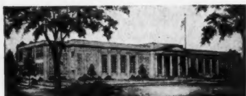
COLESTOCK HIGH SCHOOL, TITUSVILLE, PENNA. . . ARCHITECT—W. Holmes Crosby, Oil City . . . HEATING CONTRACTOR—Wm. M. Clark & Company, Inc., New Castle Webster Vacuum System
