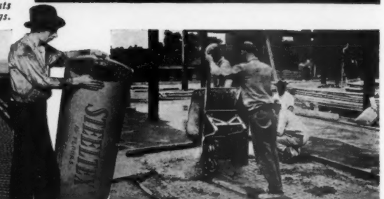
Concrete is poured directly onto STEELTEX Floor Lath. The galvanized wire reinforcing mesh is automatically embedded in the slab as the concrete is poured.
