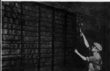
Ribbed STEELTEX Lath for plaster and STEELTEX Channels form a practical and modern method of constructing school partitions.
