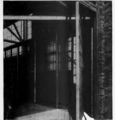
Curved Track Hangar Door
