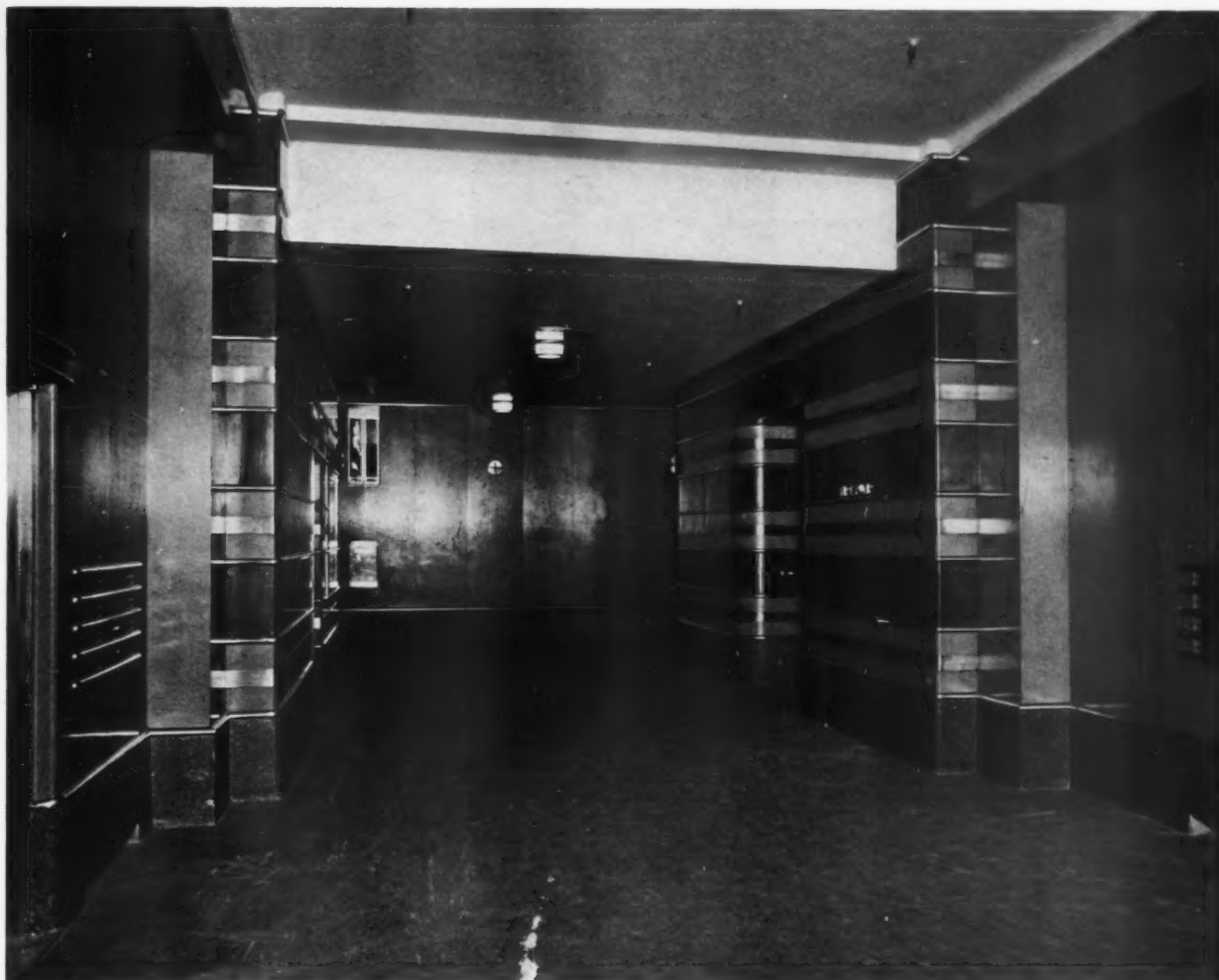
UNITY BETWEEN EXTERIOR AND LOBBY is secured by repeating the decorative scheme and colors of the entrance shown on page 29—bands of dark blue, olive green, lacquered brass and white metal
