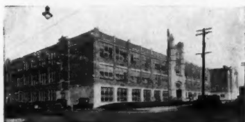
BEAVER FALLS HIGH SCHOOL, BEAVER FALLS, PENNA. . . ARCHITECT—Carlisle & Sharrer, Pittsburgh . . . HEATING CONTRACTOR—Wm. M. Clark & Company, Inc., New Castle Webster Vacuum System
