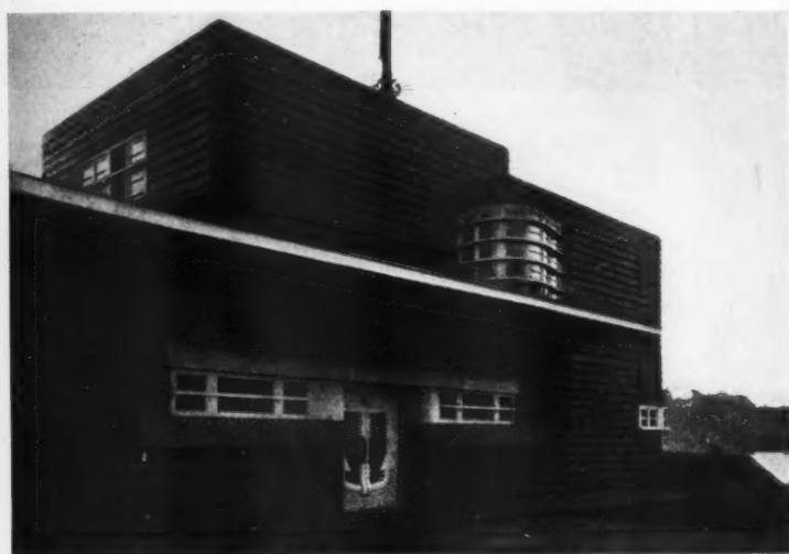
BLACK METAL-SHEATHED weather-boarding covers the walls of the Amstel Boat Club, Amsterdam, Holland, designed about ten years ago in the spirit of free yet romantic modernism by the late de Klerk, architect. From "Architect & Building News"
