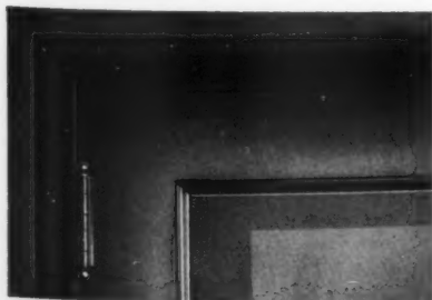
View from inside of door equipped with the new YALE Concealed Door Closer. Note the entire absence of any evidence that the door is thus controlled.
