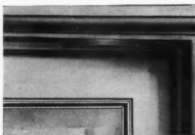
View of the same door from the outside. The only external indication of the closer is the small additional member on the trim to permit the action of the arm.
