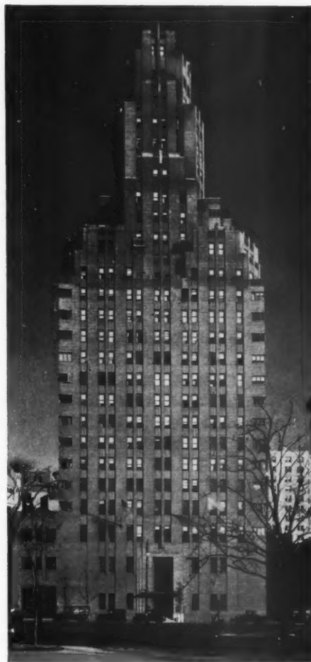
Apartment Building at Riverside Drive and 103rd St., New York City. Also housing the Roerich Museum and the International Art Center. Helmle, Corbett & Harrison, architects. Longacre Engineering & Construction Co., builders. Double Gypsum Block Partitions sound-proofed with Cabot's Quilt.
