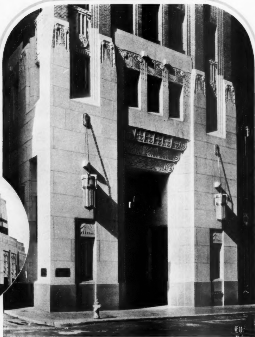
Pacific National Bank Building, San Francisco, faced and ornamented with cast stone made with Atlas White. O'Brien Bros. & W. D. Peugh, architects; Cahill Bros., general contractors, both of San Francisco. Cast stone furnished by P. Grassi & Co., Traverite Works, Inc., San Francisco.
