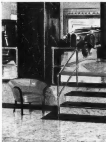
Another floor in the Chrysler showroom. A white Marble Inlaid background (Design No. 13131) set off by a black marbled border. Stair risers and treads, too, are linoleum.
