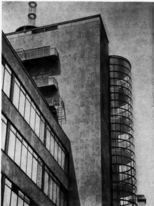
GLASS AND METAL semi-circular stair tower of the new building for E. Breuninger, Stuttgart. The design of this building, by Eisenlohr and Pfennig, is characterized by a few materials economically and effectively used in broad areas, resulting in pleasing simplicity. From "Modern Bauformen"
