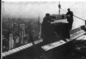
Cheney Flashing being installed on the parapet above 36th floor — Empire State. Note key-ways in flashing ready for mortar. Also the absence of dowels.
