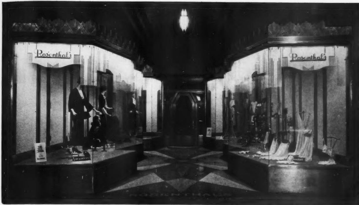
Rosenthal's Store, Chattanooga, Tenn. A Desco Store Front—installed by the Detroit Show Case Co.
