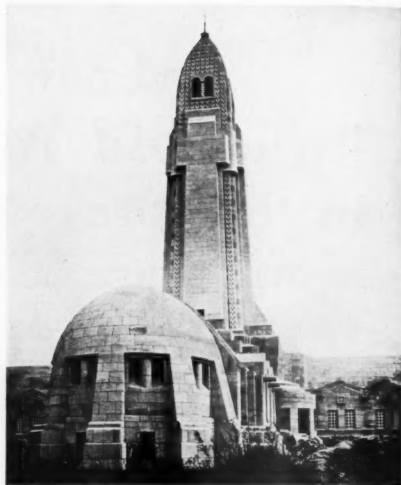
Church designed by L. Azema, M. Edrei and J. Hardy, Paris
