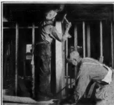
Flax-li-num insulation, water-proof building paper and metal lath plaster base, economically installed at one operation.
