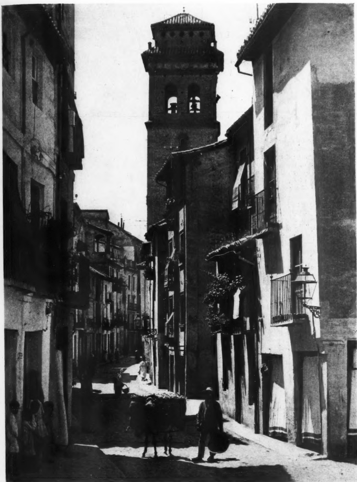
NO RAIN had fallen for seven months, yet throughout Spain, in even the most squalid locations, were found window ledges and balconies lined with flower pots. This street scene in Granada is typical of the streets in Toledo and Seville, where Moorish and Renaissance architecture has been logically combined
