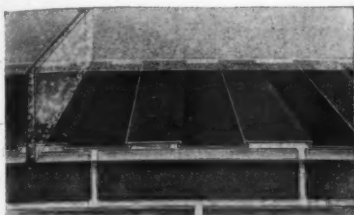
Phantom - showing Cheney Flashing under coping stones — the method employed in protecting parapet walls of the Empire State.
