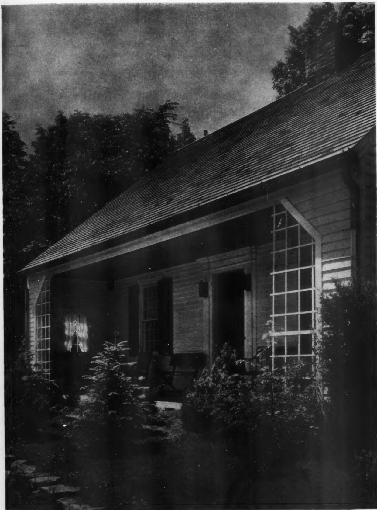
A beautiful view and the desire for something more comfortable than the conventional porch resulted in this outdoor living room, which meets the client's practical and esthetic requirements
