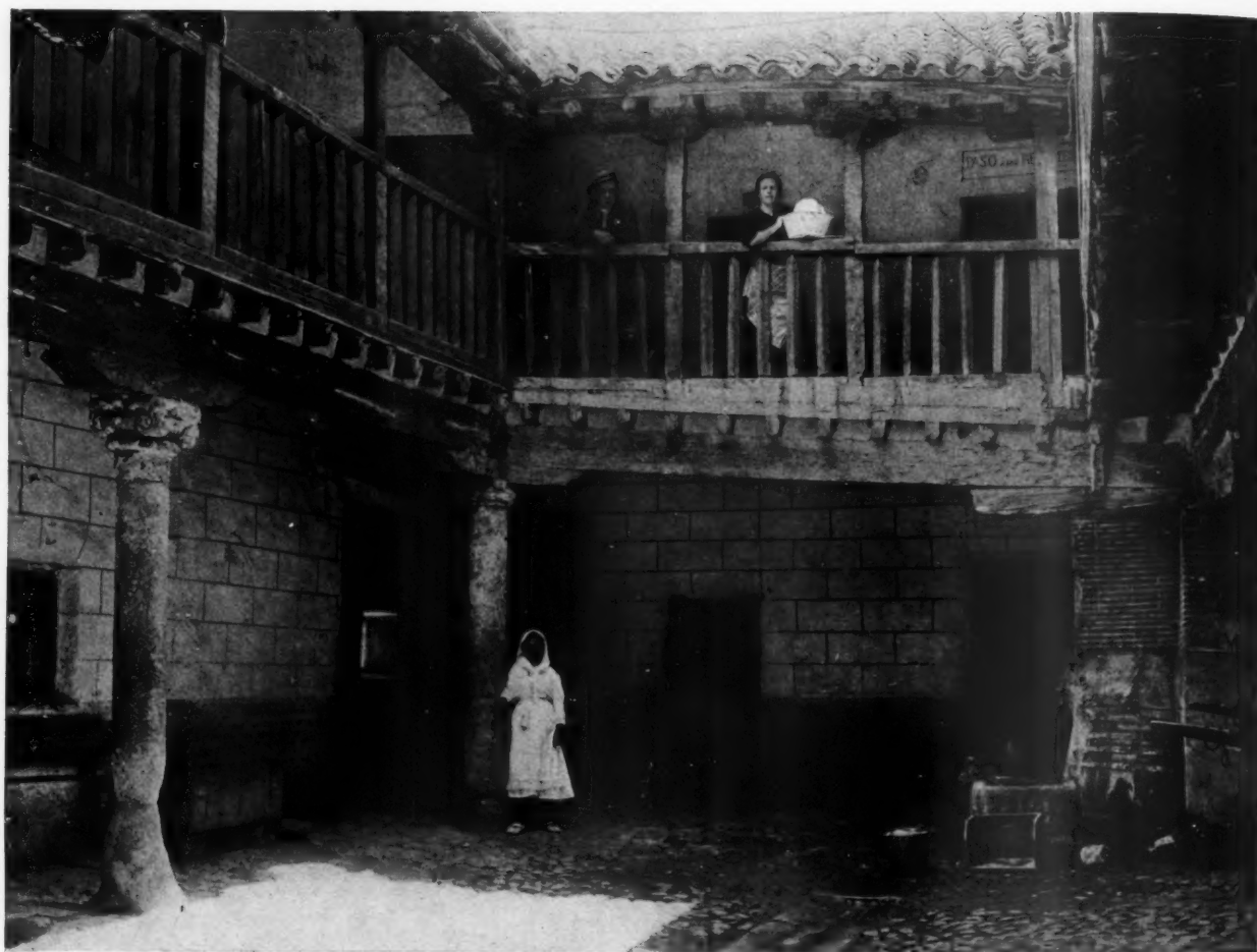
The sag in the handrail at the top is less than that of the big girder resting on the brick pier and the balcony has been built up several times. The "stone joints" are painted on stucco. In Toledo
