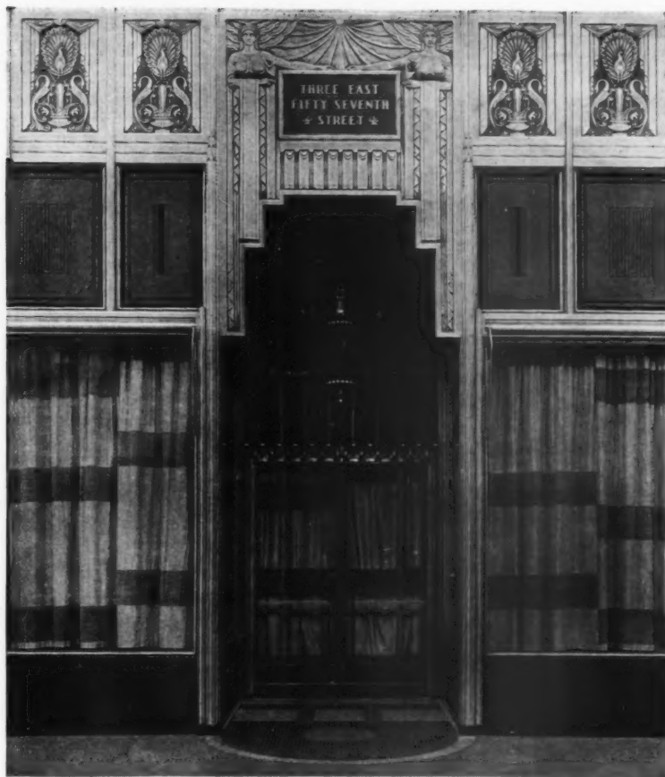
View showing the rich ornamental panels cast in Alcoa Aluminum used for main entrance. The hardware of the door is also of Alcoa Aluminum.
