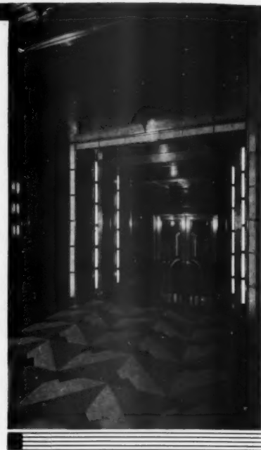
Lighted cylinders and panels contribute to the decoration and the illumination of this lobby.
