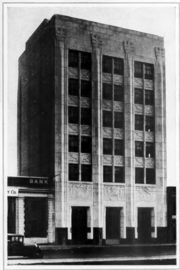
Facing of cast stone on the Income Securities Building, Oakland, Calif. F. H. Reimers, Oakland, Calif., architect; C. W. Heyer, Jr., San Francisco, general contractor. Cast stone, made with non-staining Atlas White portland cement, furnished by Stonetex Corporation, San Francisco.
