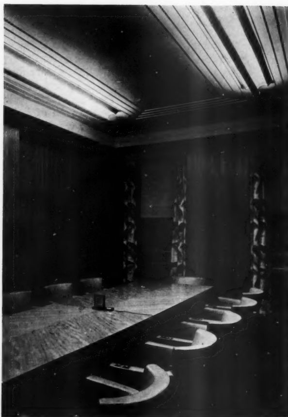
DIRECTED-INDIRECT principle of lighting as applied in this room gives clear, even illumination where most desirable
