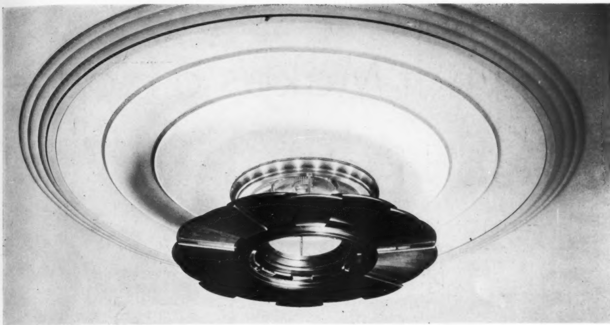
METAL LOUVRES conceal the lamps and reflect the light against a plaster rosette designed to spread light over the entire area. Directed - indirect principle
