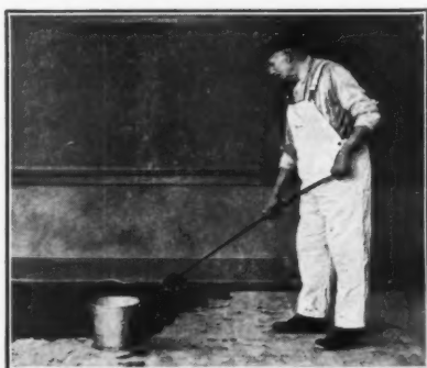
Lignophol is easily and quickly applied with a long-handled brush.
