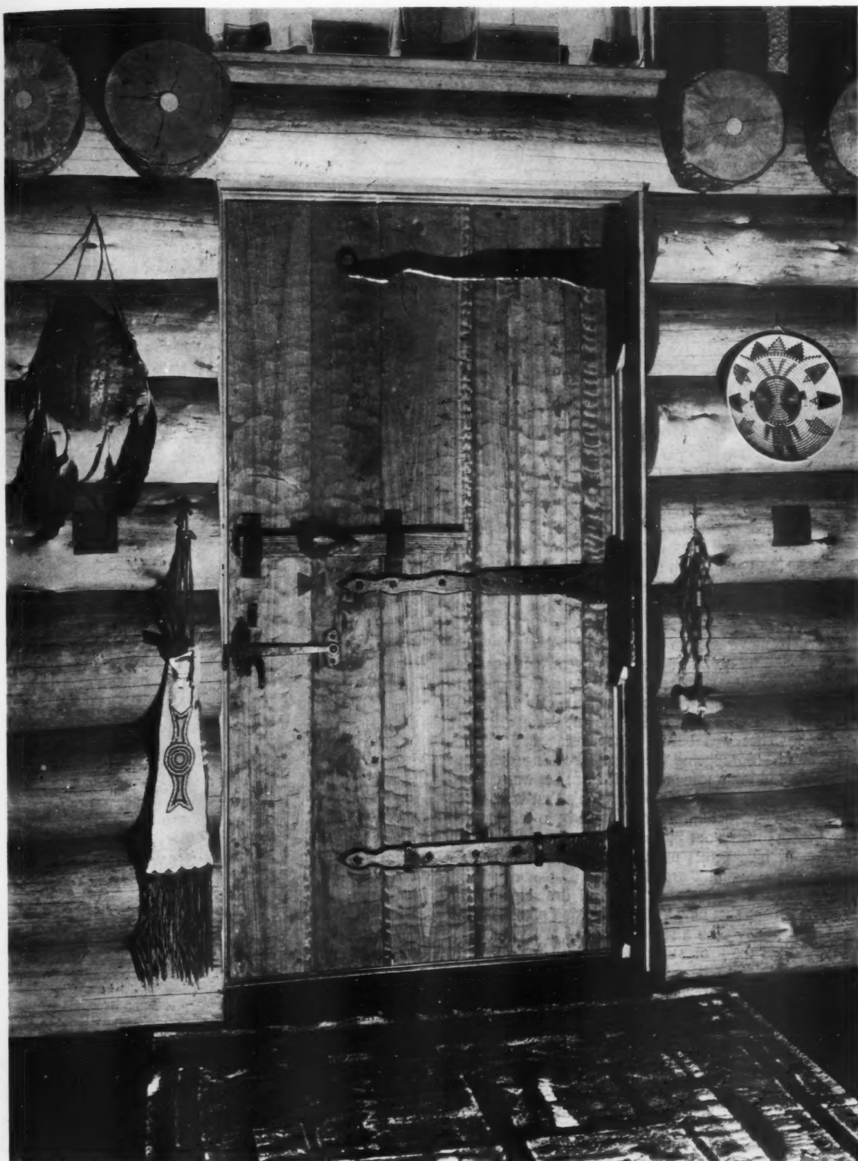
HAND FORGED hardware, plank door, plank floor, and logs stripped of bark give to the entrance vestibule a suggestion of the exterior
