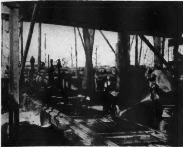
THIRTY-INCH trees could be cut on this circular saw installed on the job
