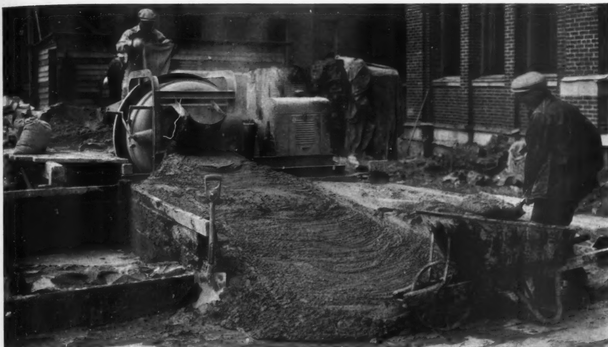
Mixing Mortar for the Lane Technical High School, Chicago
