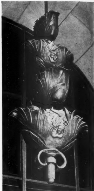
INDIRECT illumination using a fixture based upon the architecture of which it is a part. Use is made of walls of the entrance as reflecting surfaces
