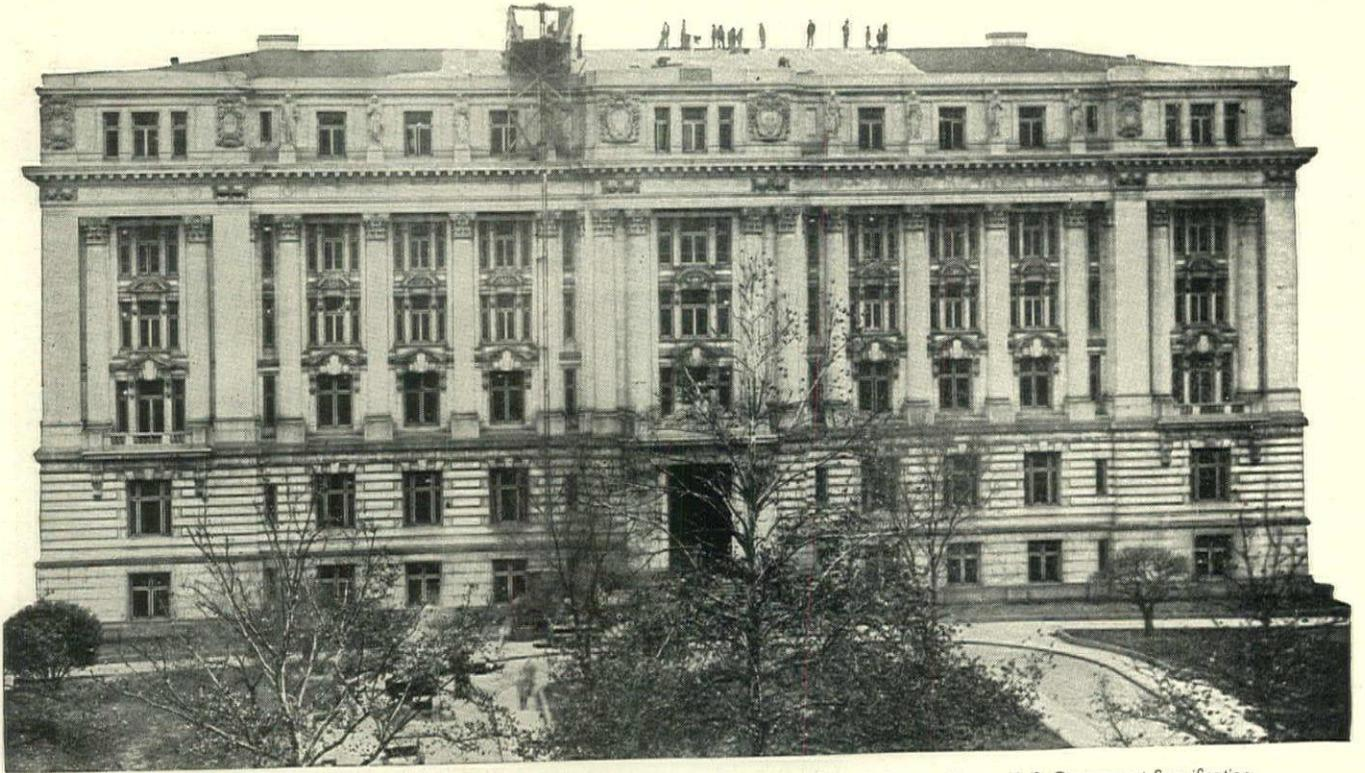
Reroofing the District Building, Washington, D. C., with a Carey 5-ply Feltex Built-Up Roof, applied according to U. S. Government Specification
