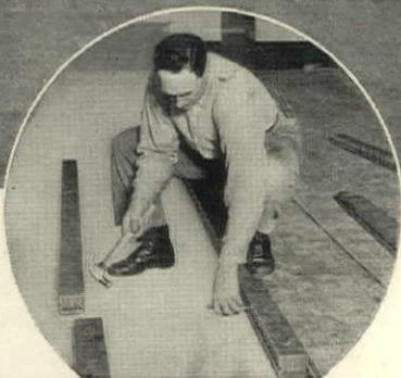
Bloxonend is furnished in 8 foot flooring lengths. The tough end-grain forms the wearing surface.
