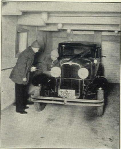
FORTY BELOW ZERO tests Carter Carburetor operation here, thanks to Armstrong's Corkboard on the walls and Cork Covering on the cold lines.
