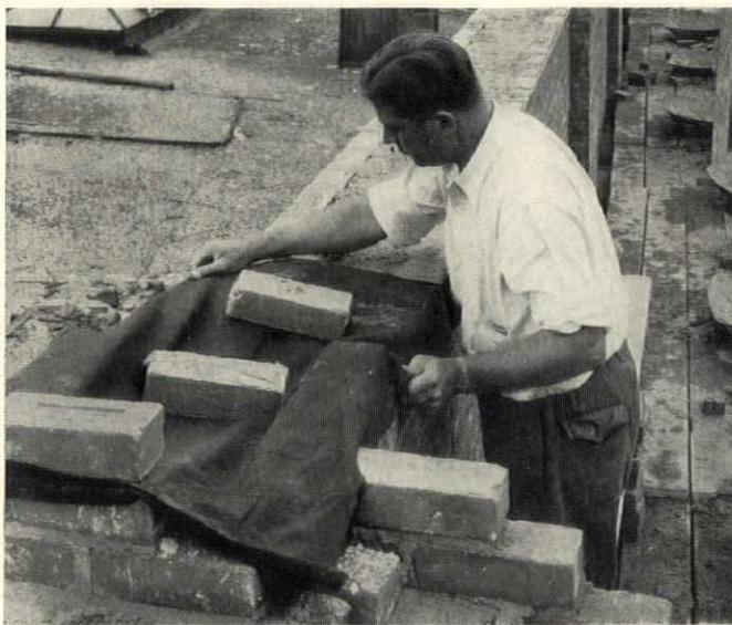
*PROTECTING WORK against rain or heavy dew. At quitting time work is left stepped for good bonding*
