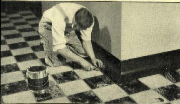
Picture shows mechanic completing the job, spreading linoleum paste under edge of the border and the patterned linoleum used for the floor.
