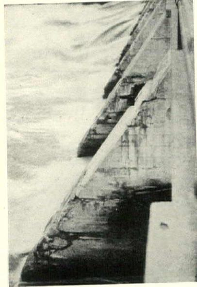
How excess water causes disintegration. From "Basic Principles of Concrete Making"
