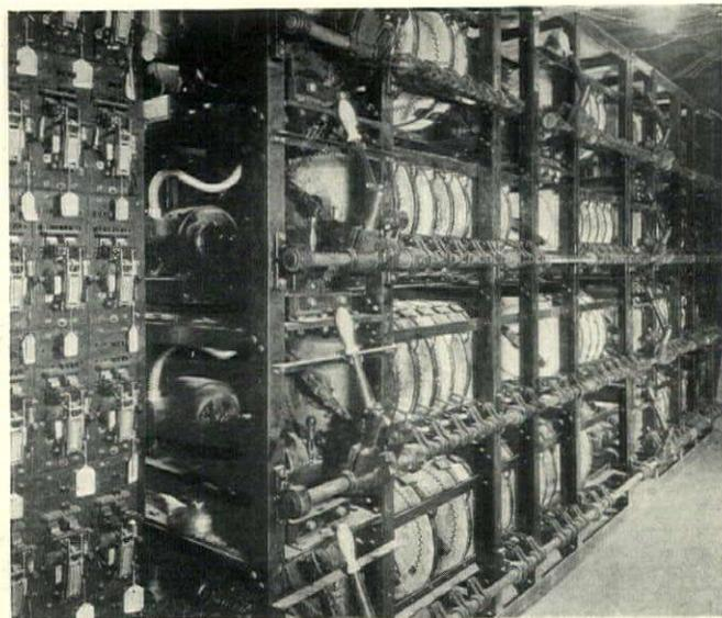
Part of switch board and dimmer bank, which can be operated by one man from a single control board
