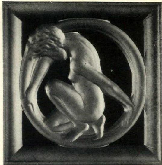
*Perforated ventilating grille of moulded glass designed by Frederick Carder. The units are about eight inches square*
