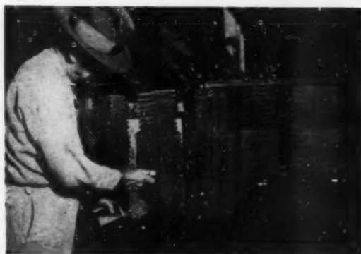
GRADE MARKING LUMBER ACCORDING TO AMERICAN LUMBER STANDARDS
