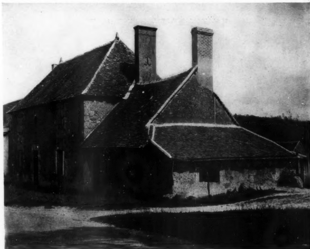
VARIETY IN ROOF TREATMENT AND PROPORTION OF INDIVIDUAL MASSES LEND A PICTURESQUENESS TO THIS FARM HOUSE IN GRAND VALLEY, FRANCE
