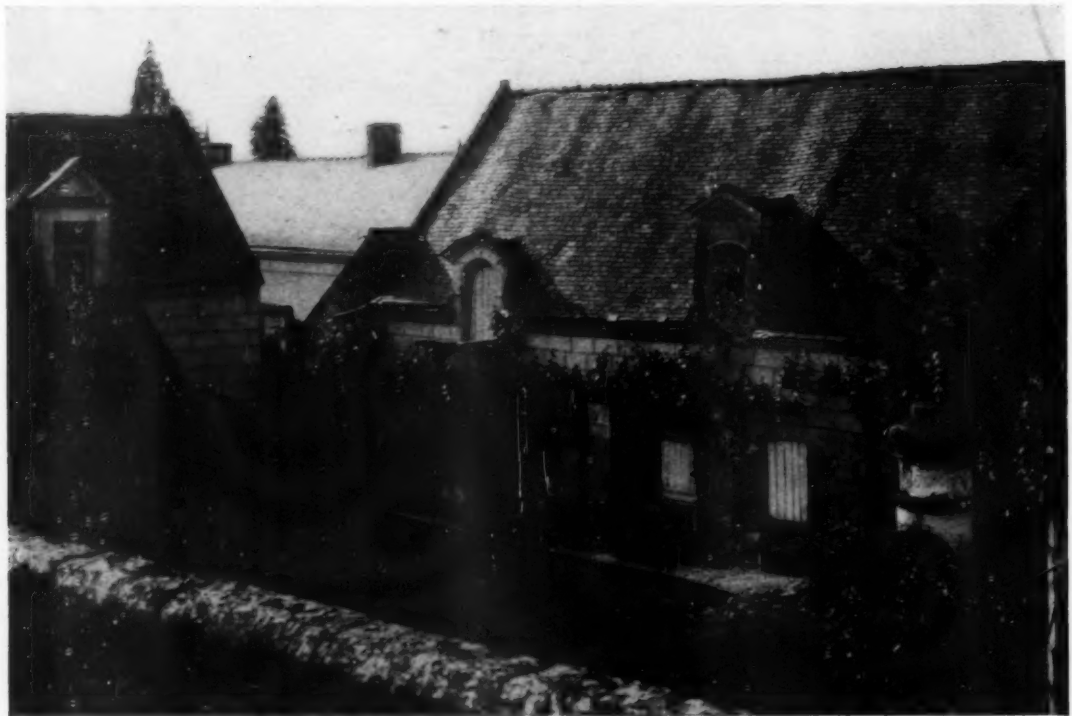
COURT GROUP ON BANKS OF LOIRE RIVER NEAR LA BOHALLE, FRANCE IN BOTH ENGLAND AND FRANCE PICTURESQUE INFORMALITY IS FOUND WITHOUT LOSS IN DIGNITY
