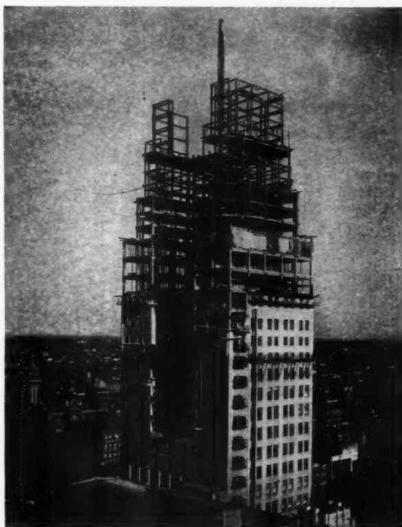
KANSAS CITY ADMINISTRATION AND EQUIPMENT BUILDING. SOUTHWESTERN BELL TELEPHONE CO., KANSAS CITY, MO.
