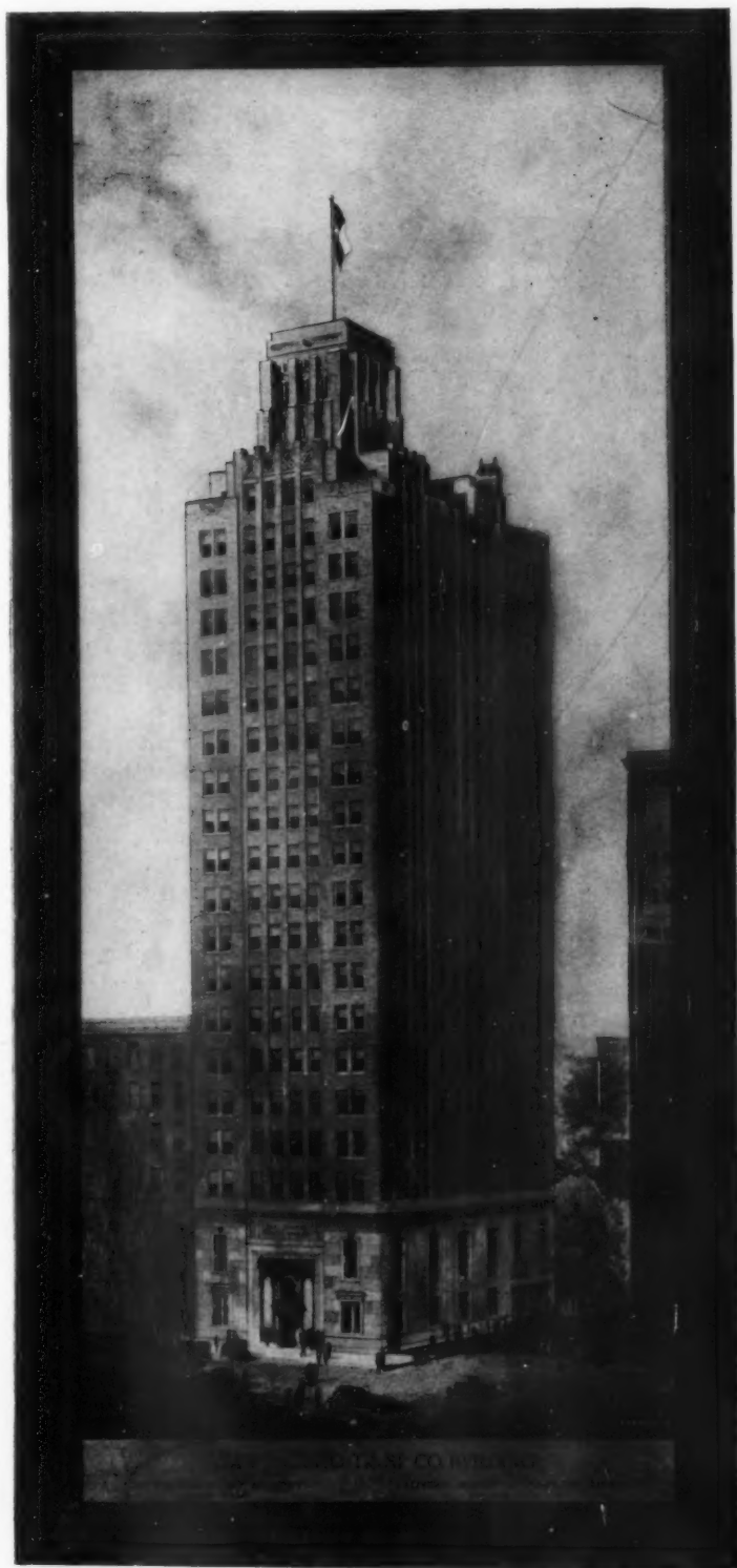
SAN JACINTO TRUST COMPANY BUILDING, HOUSTON, TEXAS JOS. W. NORTHROP, ARCHITECT—ALFRED C. BOSSOM, CONSULTING ARCHITECT
