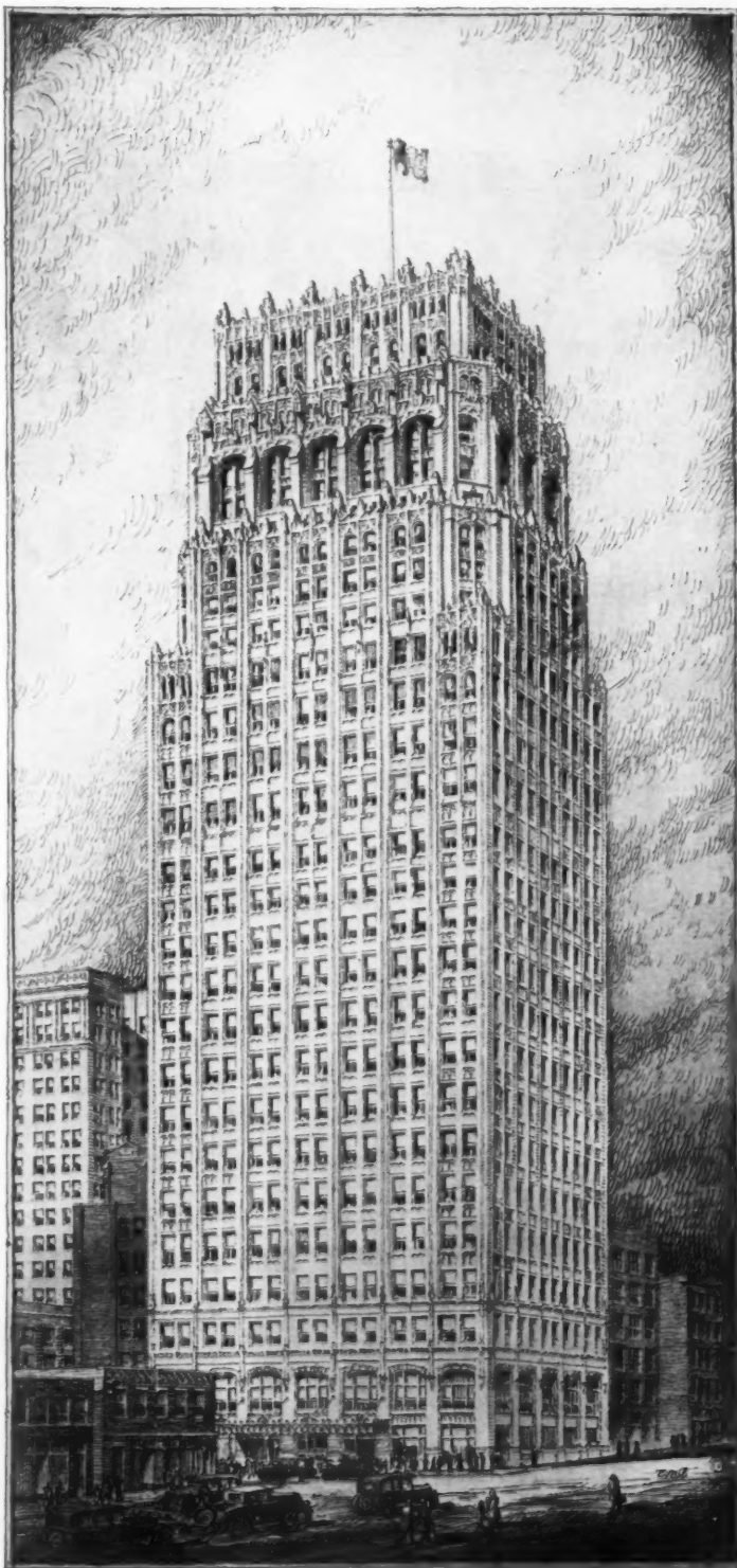
KANSAS CITY ADMINISTRATION AND EQUIPMENT BUILDING, SOUTHWESTERN BELL TELEPHONE CO., KANSAS CITY, MO.
