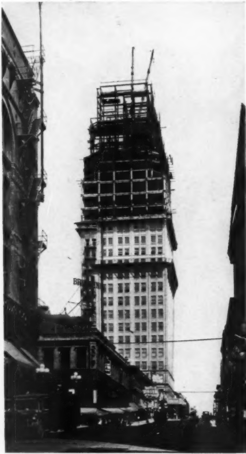
KANSAS CITY ADMINISTRATION AND EQUIPMENT BUILDING, SOUTHWESTERN BELL TELEPHONE CO., KANSAS CITY, MO.
