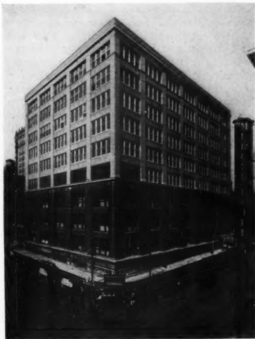
ARGYLE BUILDING, KANSAS CITY, MO. KEENE & SIMPSON, ARCHITECTS
