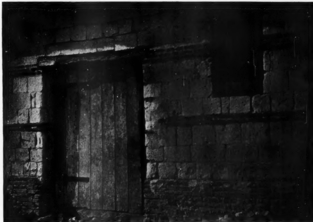
OLD BARN AT FERME DE TOUPTS, NORMANDY A WALL OF ALTERNATE BANDS OF BRICK AND CHALK
