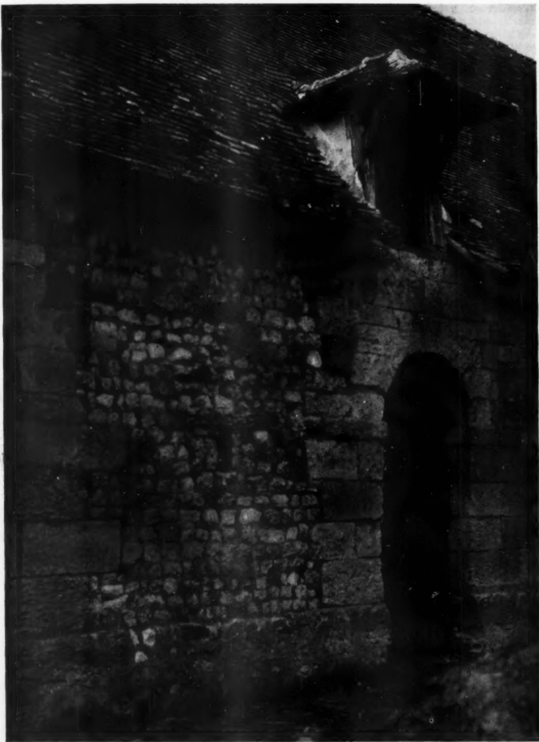
DETAIL OF AN OLD FARM BUILDING AT QUEVILON
