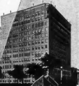
BERKMAN-BROOKHUIS APARTMENT BLDG. Architect: Blumen & Hensel Electrical Contractor: U.M. Electric Co.
