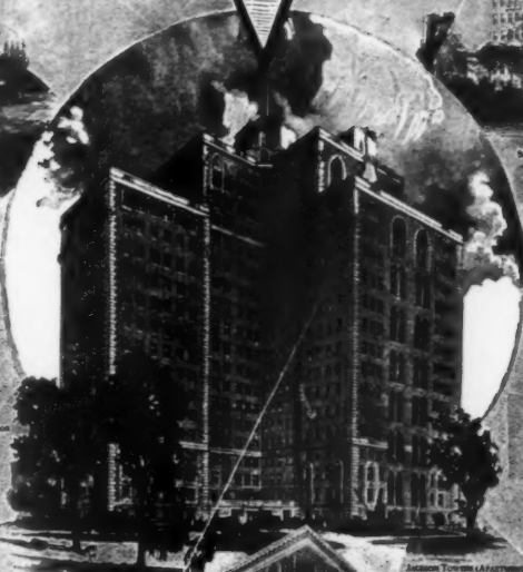
JACKSON TOWER (Apostrophe Hotel) Architect: Walter W. Johnston Electrical Contractor: Wan & Tully Electric Co.
