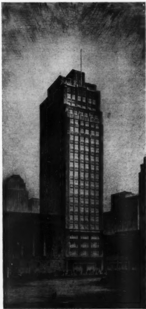
LEFCOURT-EMPIRE BUILDING, NEW YORK BUCHMAN & KAHN, ARCHITECTS
