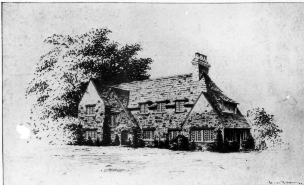
HOUSE IN SCARSDALE, NEW YORK—HAROLD BROWN, ARCHITECT
