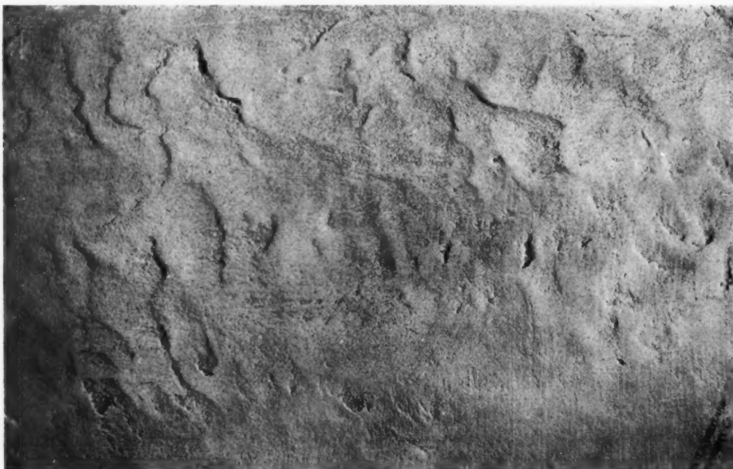
AFTER APPLYING THE PLASTIC PAINT EVENLY WITH A BRUSH, THE LAPS WERE OBTAINED BY A SLIGHT WRIST MOVEMENT WITH THE SAME BRUSH, PARTLY DRY. THE PECULIAR SLIGHT ROUGHNESS IN THE TEXTURE, AS NOTICEABLE IN THE CENTER OF THE PANEL, IS THE RESULT OF "SKIPPING" WHEN USING THE BRUSH
