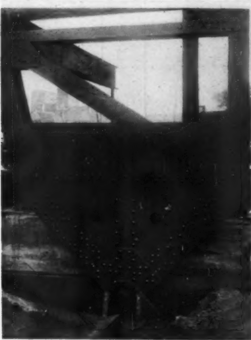
PIN CONNECTION AT BOTTOM OF TRUSS
