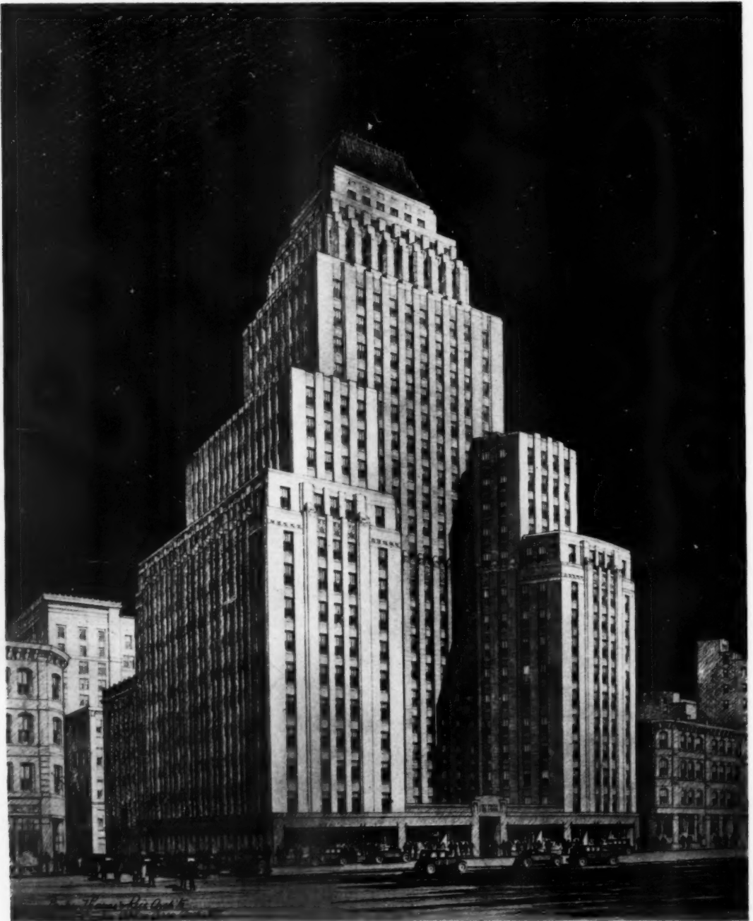
UNITED SHOE MACHINERY CORPORATION BUILDING, BOSTON, MASS. PARKER, THOMAS & RICE, ARCHITECTS; HENRY BAILEY ALDEN, ASSOCIATE ARCHITECT
