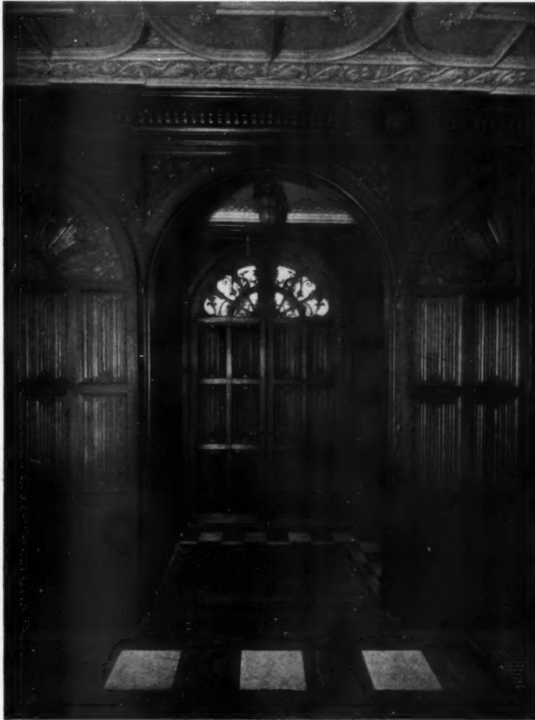
THE SPECIAL WOODWORK IN THE RESIDENCE OF MR. PAUL WATKINS
