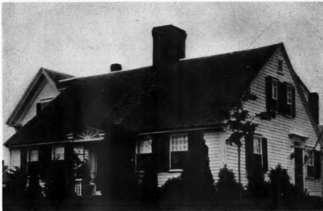
OLD HOUSE ON ROAD NEAR HYANNIS, CAPE COD, MASS.
