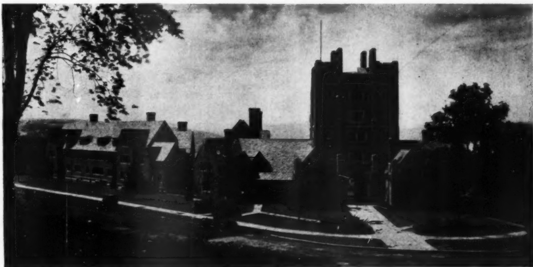
BAKER TOWER AND FOUNDER'S HALL FROM WEST AVENUE
