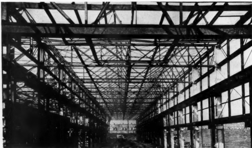
INTERIOR OF NORTHERLY AISLE OF GENERAL ELECTRIC COMPANY BUILDING AT WEST PHILADELPHIA, PA., IN WHICH STRUCTURAL MEMBER CONNECTIONS ARE WELDED
