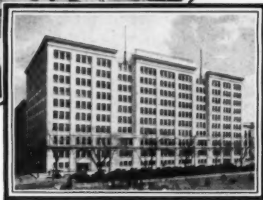
Architects: A. E. Harrison and H. W. Wagner, Santa Fe System, Chicago. General Contractors and Plasterers: Swenson Construction Co., Kansas City
