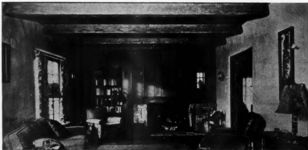
HOUSE AWARDED FIRST PRIZE IN THE 1927 COMPETITION CONDUCTED BY THE WEST COAST LUMBER BUREAU, AS BUILT. CEILING AND FLOOR OF LIVING ROOM ARE OF WIDE RANDOM WIDTH DOUGLAS FIR. CEILING BEAMS ARE SAND ETCHED
