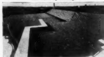
Finished roof of the Jefferson Vocational School where this double use of Insulite was so successfully worked out.
