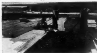
Steel roof deck is applied over Wall Board sheets and then covered with 1/2" Insulite Roof Insulation, over which is mopped the first felt of standard built-up roofing.
