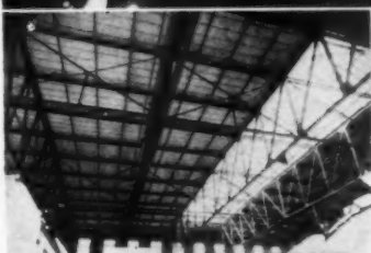
Under side of roof, showing sheets of Insulite Wall Board exposed for acoustical correction. Natural finish of Insulite makes a most attractive appearance.
