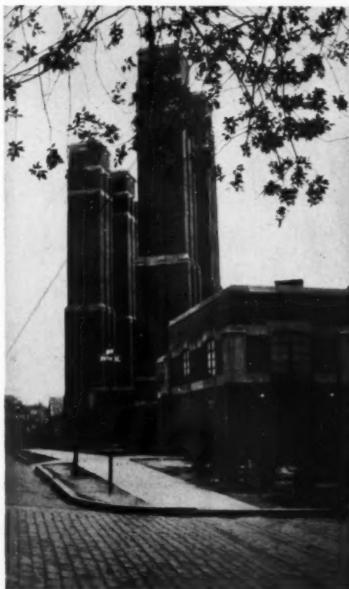
THE PAIR OF TWIN TOWERS OF THE LIBERTY TUNNEL FAN HOUSE ARE THE PRINCIPAL ARCHITECTURAL FEATURES
