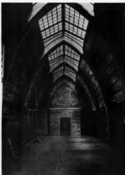
A SKYLIGHT PROVIDES NATURAL ILLUMINATION
