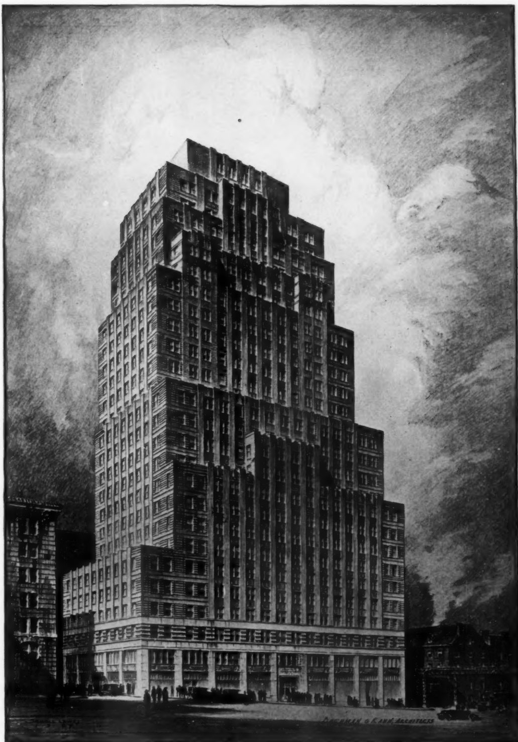
INSURANCE BUILDING, NEW YORK—BUCHMAN & KAHN, ARCHITECTS
