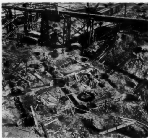
TOWER AND CHUTES USED IN PLACING CONCRETE
