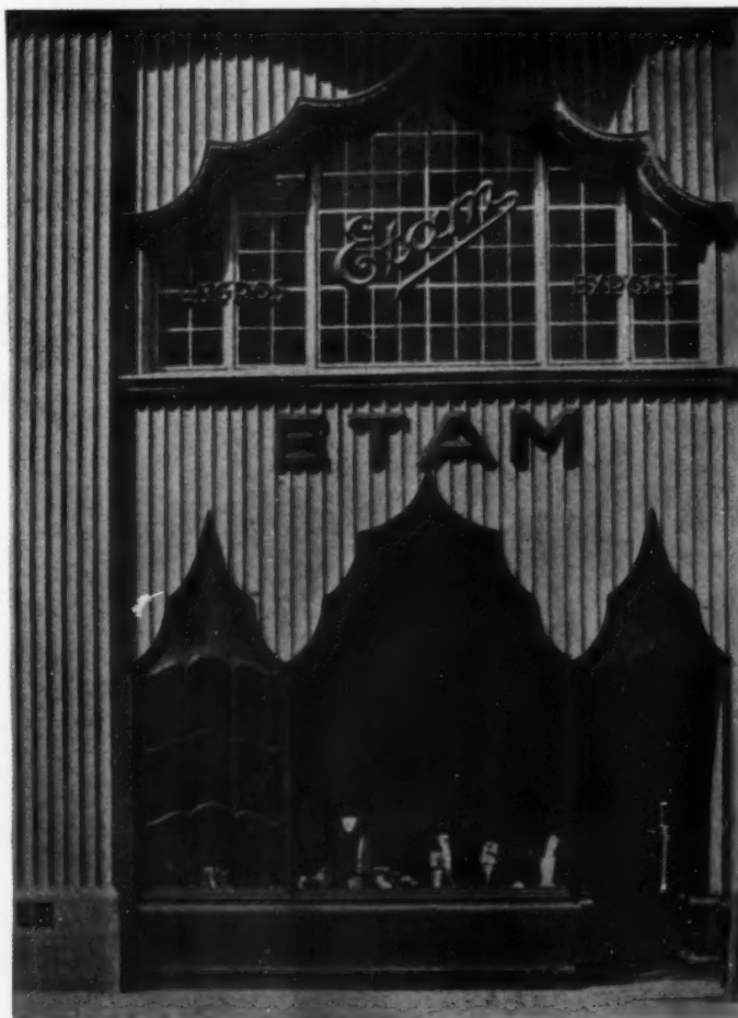
INTERESTING FRONTAGE OF HOSIERY SHOP IN THE FRIEDRICHSTRASSE, BERLIN—PAUL ZUCKER, ARCHITECT (Courtesy of "Shop Fronts")
