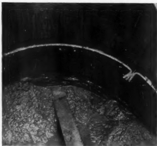
BOTTOM OF PARTIALLY EXCAVATED CAISSON
