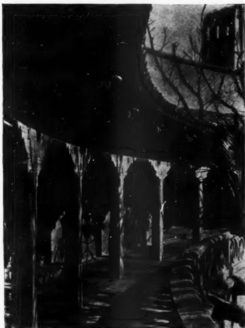
SECOND STORY OF PATIO LOGGIA
