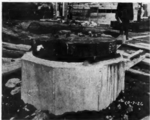
TOP OF CAISSON SHOWING STEEL BILLET SUPPORTED ON STEEL ANGLE SHIMS BEFORE GROUTING
