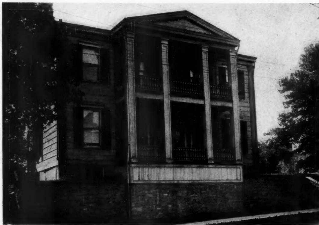
HOUSE ON CALIFORNIA AVENUE, ST. LOUIS, MO.—ABOUT 1850
