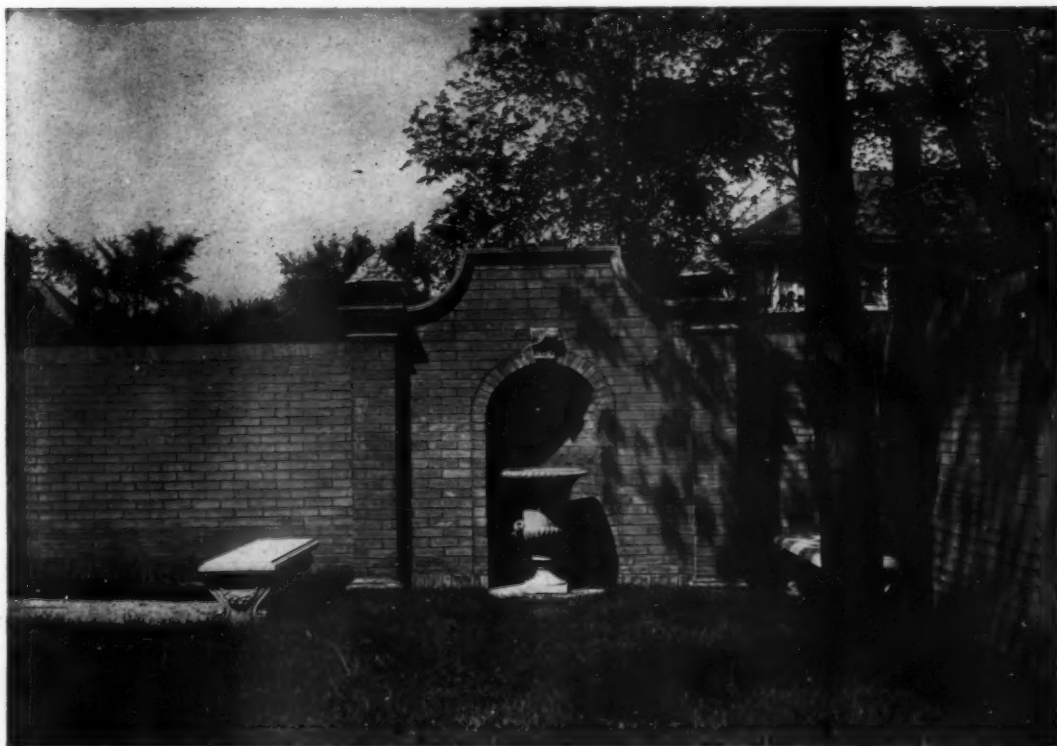
GARDEN DETAIL, HOUSE OF A. G. MILLER, ST. LOUIS, MO.—JOHN ALBURY BRYAN, ARCHITECT
