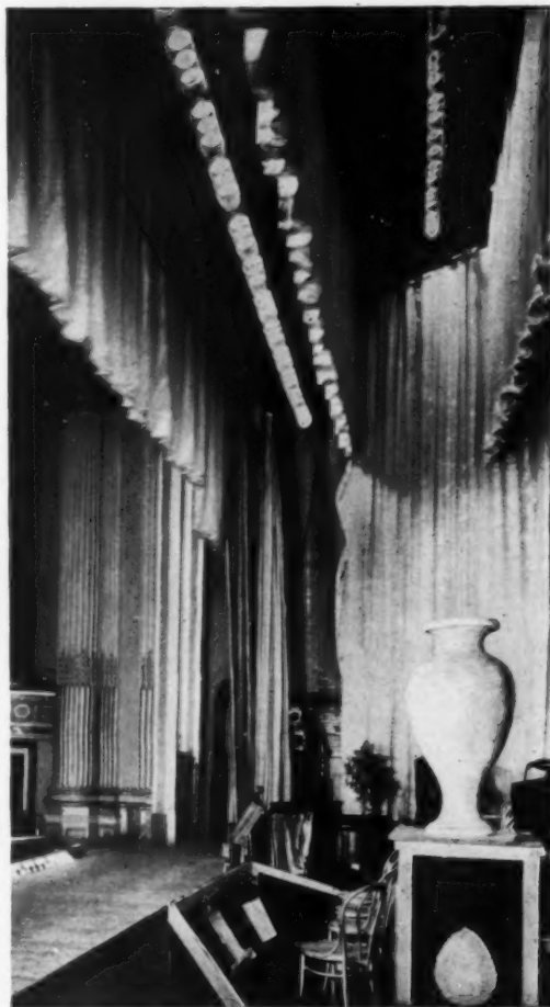
PARK THEATRE, CLEVELAND—PAUL LAMB, ARCHITECT FOOTLIGHTS AND BORDERLIGHTS OF THE INDIVIDUAL-REFLECTOR TYPE PROVIDE THE PRINCIPAL ILLUMINATION FOR THIS "PRESENTATION" STAGE
