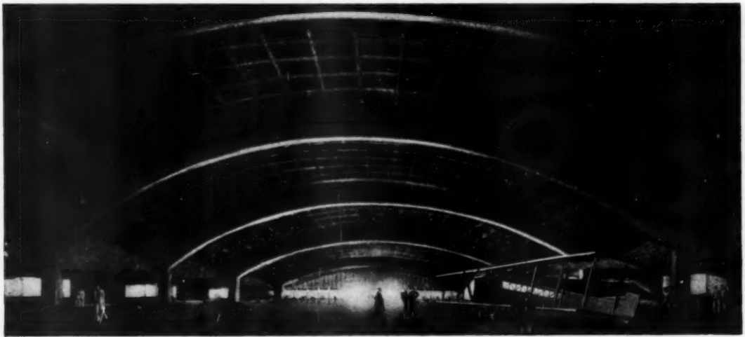
HANGAR IS 370 FEET WIDE AND 260 FEET LONG
