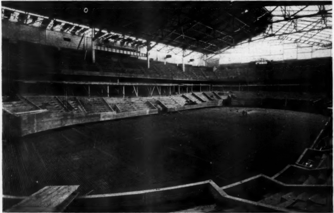
ICE SKATING FLOOR PRIOR TO POURING THE CONCRETE SURFACE SHOWING THE REFRIGERATING PIPING UNDER THE ARENA FLOOR. THE PIPING SYSTEM SHOWN REQUIRED 74,880 FT. OF 1 1/4 INCH PIPE. BUILDING CONTAINS 7,229,000 CUBIC FEET AND HAS A FLOOR AREA OF 77,393 SQ. FT.
