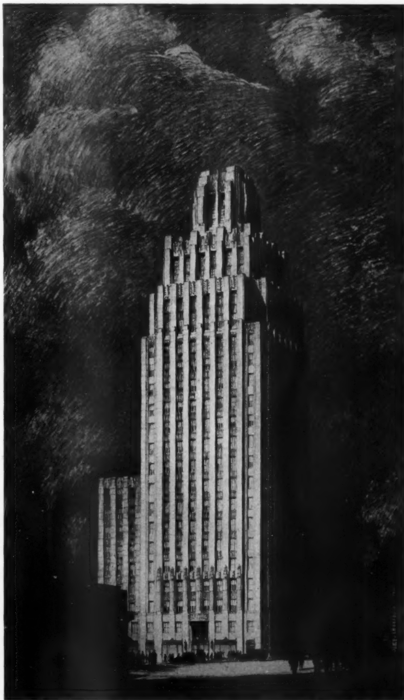
OFFICE BUILDING FOR R. J. REYNOLDS TOBACCO COMPANY, WINSTON-SALEM, N. C.
