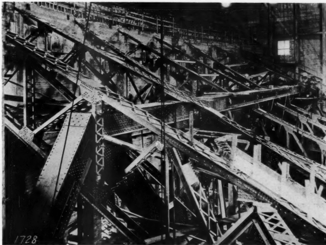
MAIN BALCONY TRUSS AND CANTILEVERS. CANTILEVERS WERE HOISTED TO CAMBERED POSITION. HOLES WERE DRILLED AND MATCHED BEFORE RIVETING. NOTE PIN JOINTS IN UPPER CHORD
