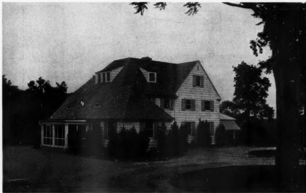
Photo by Gottscho
