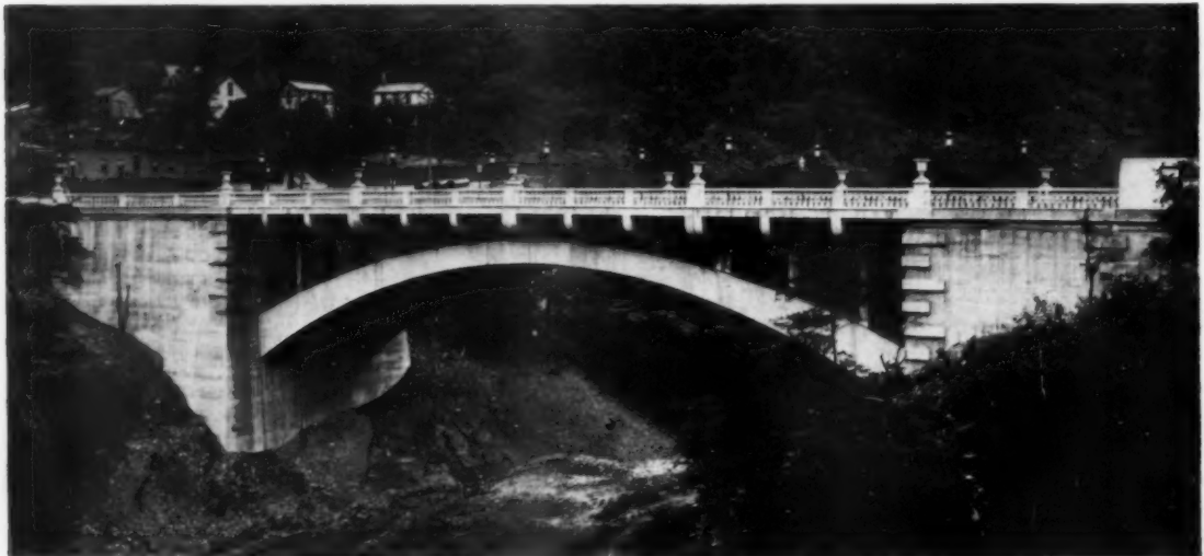
HETHS RUN BRIDGE, ENTRANCE TO HIGHLAND PARK, PITTSBURGH, PA.
