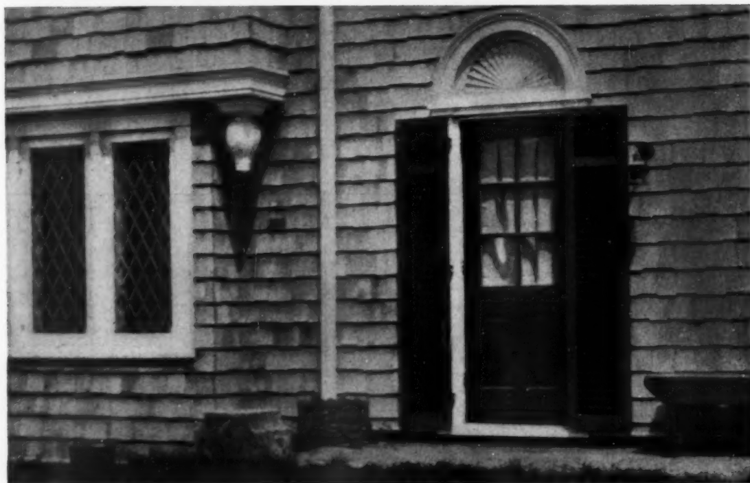
HOUSE OF FREDERIC KRULL, INDIANAPOLIS, IND. BURNS & JAMES, ARCHITECTS
