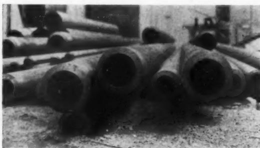
PIPE DELIVERED TO JOB WITH BEVELED ENDS
