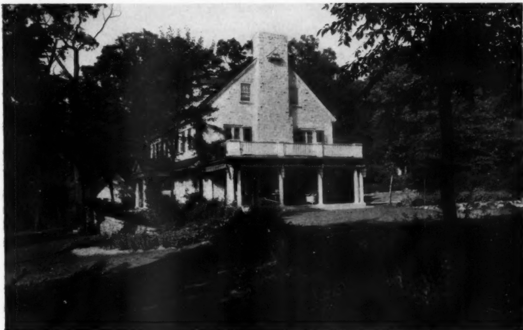
HOUSE OF MRS. FRANK HASTINGS, ALTOONA, PA. CARL A. ZIEGLER, ARCHITECT
