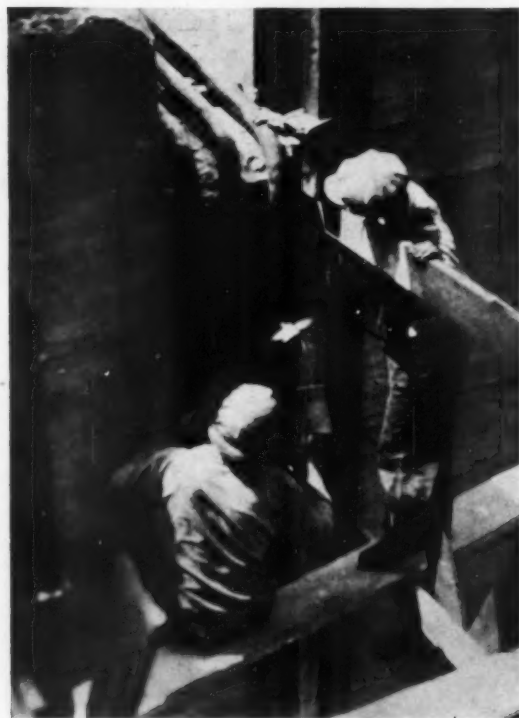
BENDS ARE MADE ON THE JOB
