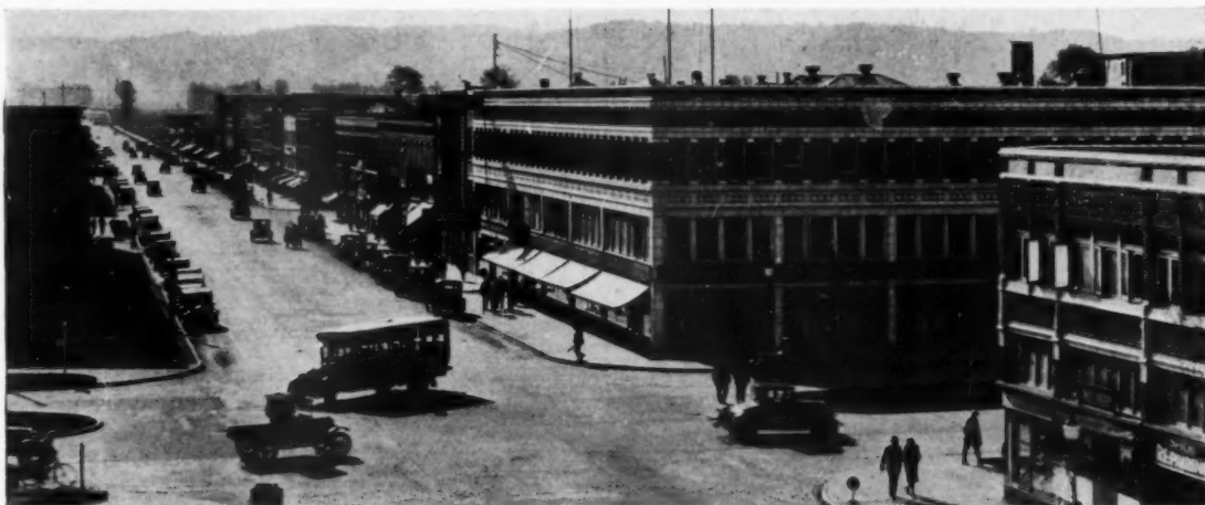
LOOKING SOUTH ON COMMERCE AVENUE, ONE OF THE MAIN BUSINESS STREETS OF THE NEW INDUSTRIAL CITY OF LONGVIEW, WASHINGTON. THE FIRST BUILDING IN THIS SECTION WAS COMPLETED IN JUNE, 1923. FOUR YEARS LATER, SIXTY-THREE MASONRY BUSINESS BUILDINGS, RANGING FROM ONE TO FOUR STORIES IN HEIGHT, WERE COMPLETED IN THIS DISTRICT, HOUSING RETAIL AND PROFESSIONAL ESTABLISHMENTS.
