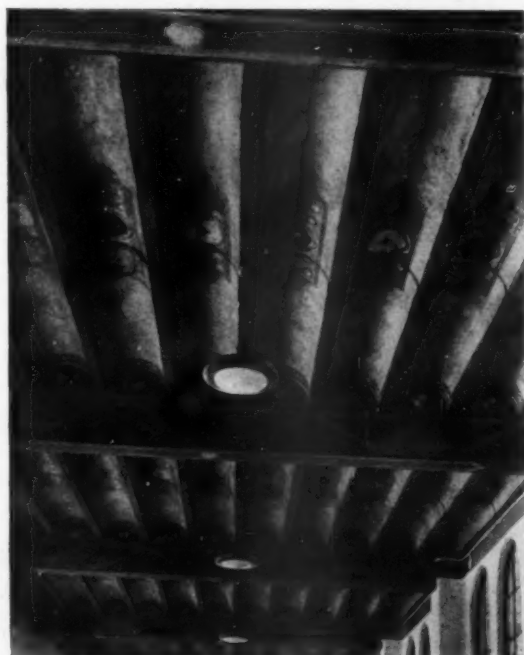
SANTA BARBARA NEWS BUILDING, SANTA BARBARA, CALIF. WASHINGTON SMITH AND EDWARD MAYBERRY, ARCHITECTS PAINTED CONCRETE CEILING OF THE MAIN OFFICE WHERE THE MARKS LEFT BY THE METAL FORMS ARE PLAINLY VISIBLE
