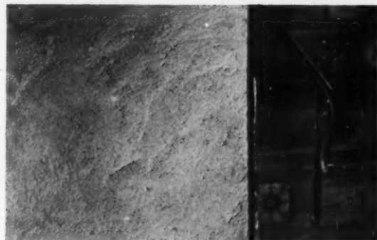
INTERIOR WALL FINISH
