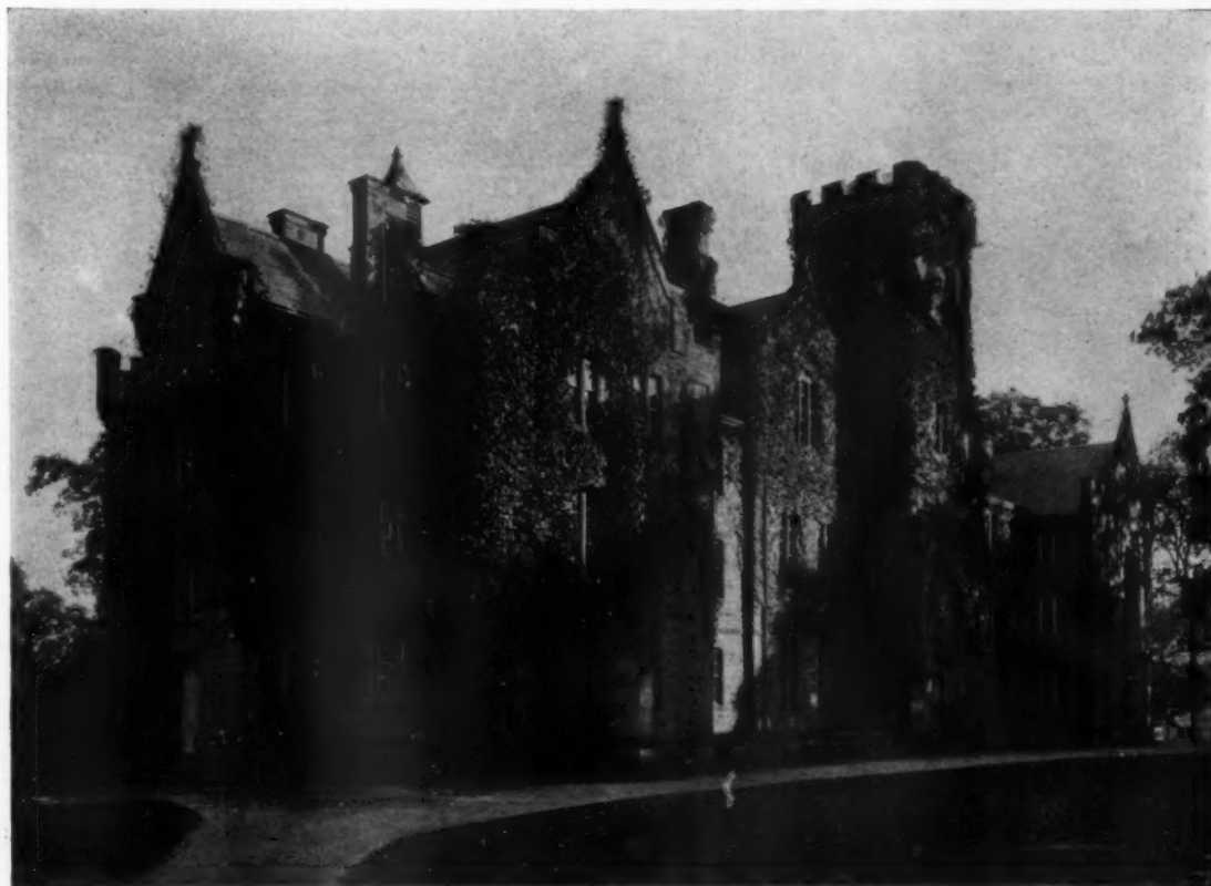
ASCENSION HALL, KENYON COLLEGE—W. TINSLEY, ARCHITECT
