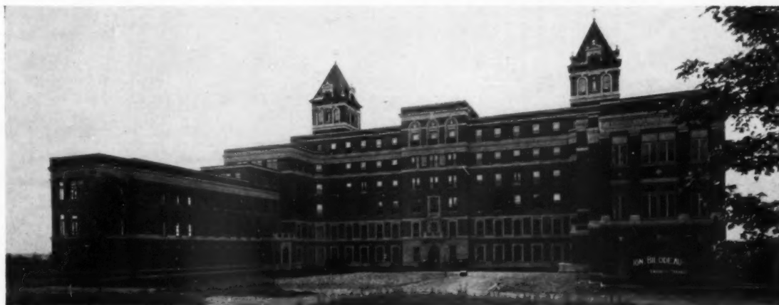
VIEW OF THE FRONT SHOWING TERRACED PAVILION EFFECT OF THE TWO MAIN WARDS OF THE HOSPITAL AND THE VENTILATING TOWERS ON THE BACK OF THE BUILDING
