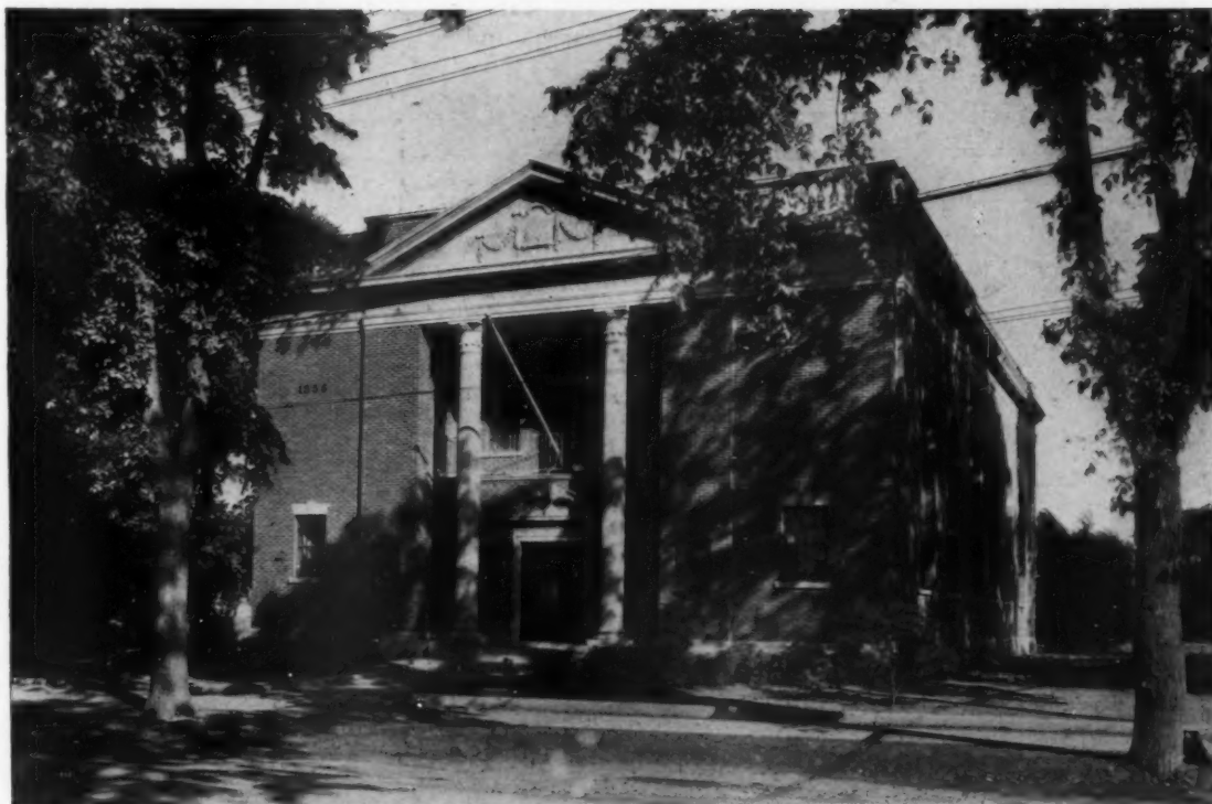
GENERAL VIEW OF EXTERIOR
