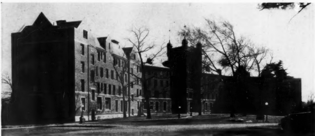
DESIGNED IN "COLLEGIATE" GOTHIC, WHICH MADE POSSIBLE A FLEXIBILITY OF FENESTRATION WHICH ADAPTED ITSELF TO THE VARYING SIZES OF OPENINGS REQUIRED IN A HOSPITAL
