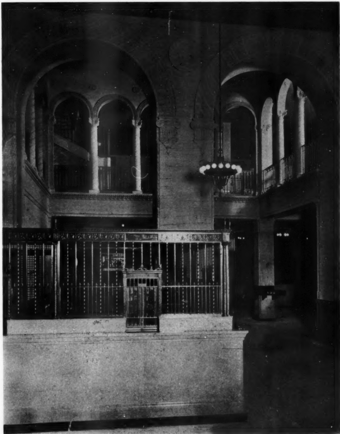
DETAIL OF BANKING SCREEN, FIRST NATIONAL BANK, TAMPA, FLA.
