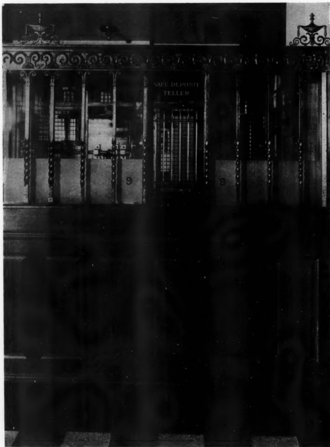
DETAIL OF BANKING SCREEN, MUTUAL TRUST COMPANY, PORT CHESTER, N. Y.
