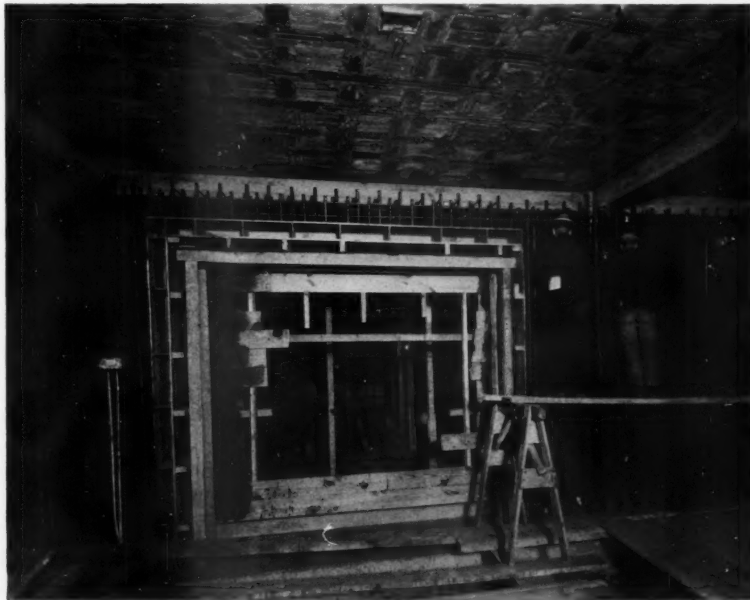
BANK VAULT REINFORCEMENT, FIDELITY-UNION TRUST COMPANY, NEWARK, N. J.
