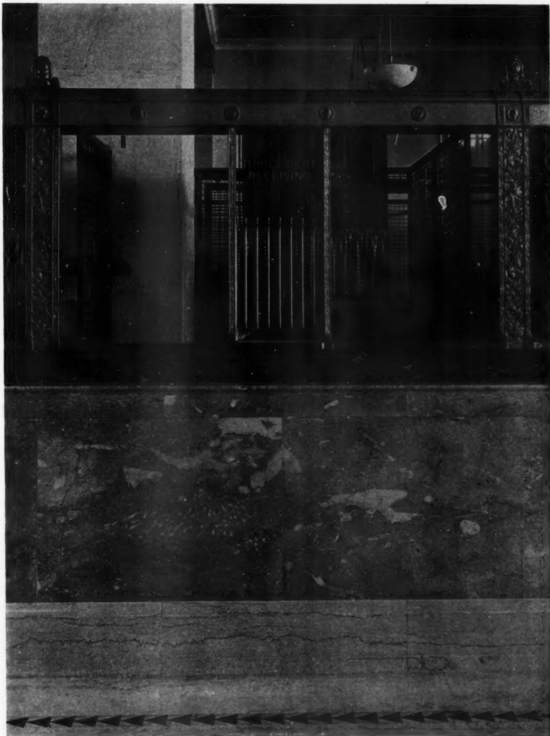
DETAIL OF BANKING SCREEN, FEDERAL TRUST COMPANY, NEWARK, N. J.
