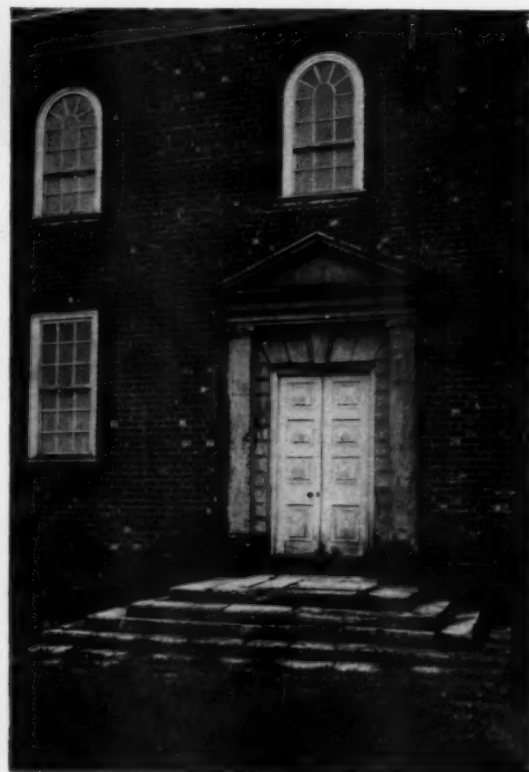
THROUGH THIS NOW SIDE ENTRANCE TO THE OLD POHICK CHURCH, WASHINGTON, ONE TIME VESTRYMAN, USED TO TAKE HIS SEAT. NOTE THE DIFFERENT COLOR OF BRICK AROUND THE FENESTRATIONS. THE SPECIFICATIONS OF THE OLD CHURCH CALL THEM "RUBBED BRICKS." THEY ARE EXACTLY THE SAME BRICKS AS THE BALANCE OF THE CHURCH, BUT BY RUBBING ONE BRICK ON THE OTHER, THE COLOR WAS INTENSIFIED
