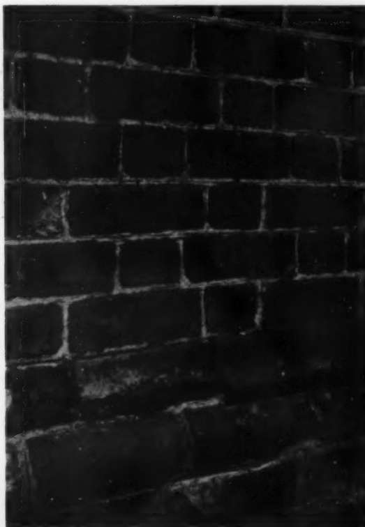
CLOSE-UP VIEW OF BRICKWORK OF OLD POHICK CHURCH. ALL THE BRICKS WERE MOULDED AND BURNED RIGHT ON THE GROUND, EXCEPTING ONLY THE WATER TABLE ONES. RUMOR HAS IT, THEY CAME "FROM DOWN RICHMOND WAY." THESE BRICKS ARE ALL 9 INCHES LONG AND 1/2 INCH HIGHER THAN PRESENT DAY ONES. THE JOINTS ARE MADE FROM A MIXTURE OF ONE PART LIME AND 3 PARTS SAND. IF YOU EXAMINE IT WITH A MICROSCOPE YOU WILL SEE THAT RIGHT THROUGH THE CENTER OF THE JOINTS THE TROWEL POINT HAS BEEN DRAWN. THIS GIVES A ROUNDED EFFECT TO THE JOINT
