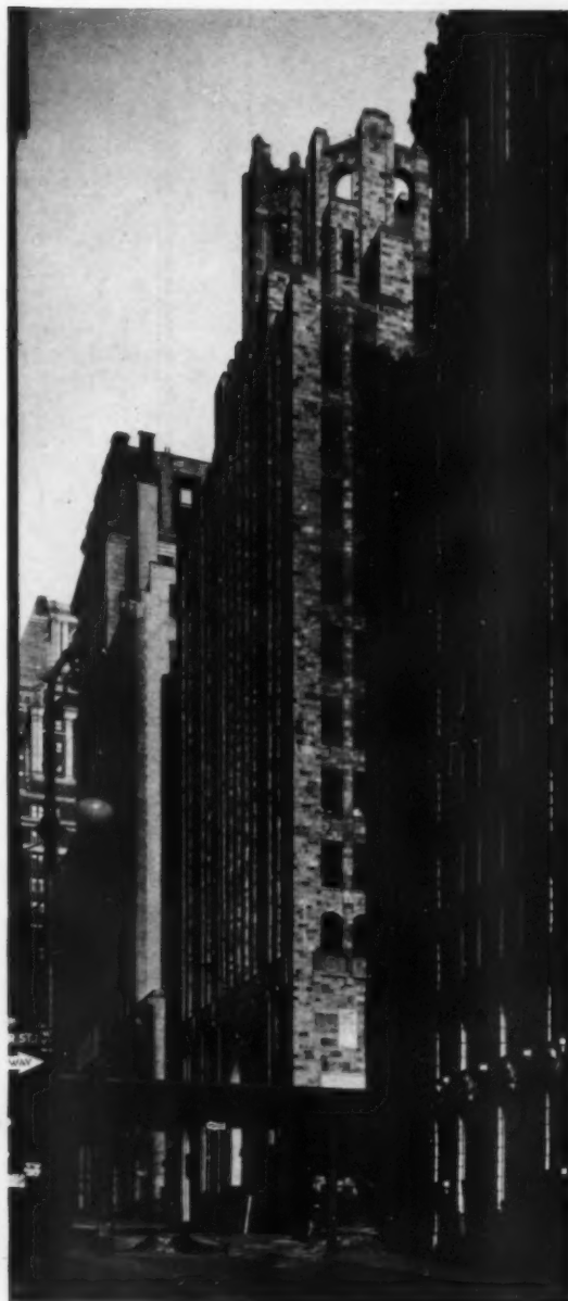
SEAMEN'S BANK FOR SAVINGS, NEW YORK BENJAMIN WISTAR MORRIS, ARCHITECT
