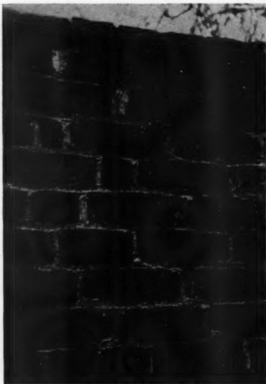
CLOSE-UP VIEW OF ONE-BRICK-THICK SERPENTINE WALL, AT UNIVERSITY OF VIRGINIA, CHARLOTTESVILLE. NOTE THE SIZE OF THE BRICKS. THEY ARE HALF AN INCH HIGHER THAN OUR PRESENT DAY STANDARDS. YOU SEE THIS GIVES A SQUARISH EFFECT TO THE HEADERS
