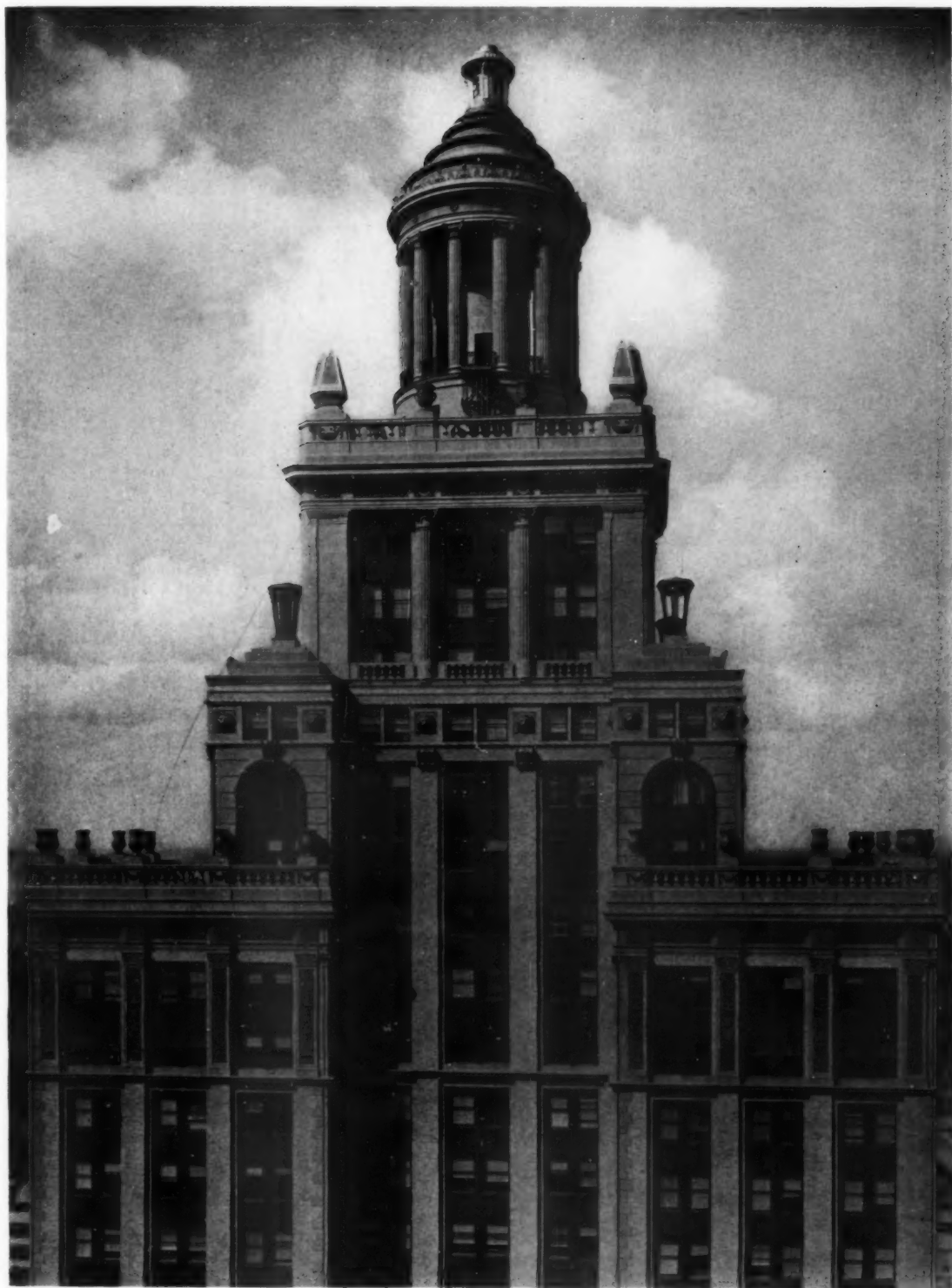
NIELS ESPERSON BUILDING, HOUSTON, TEXAS
