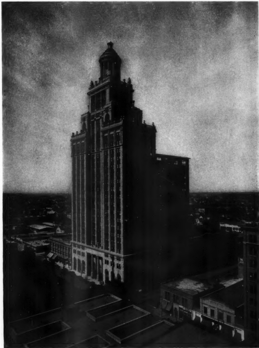
NIELS ESPERSON BUILDING. HOUSTON. TEXAS
