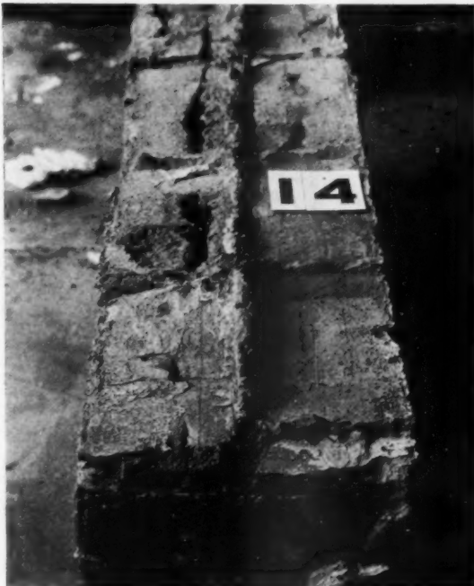
WALL NO. 14 AFTER TEST. BRICKS HAVE BEEN REMOVED TO SHOW TYPICAL BEDDING AS LAID BY MASON A
