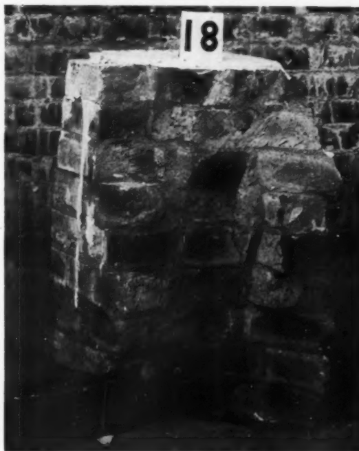
BROKEN PORTION OF WALL NO. 18 LAID WITH "SHOVED" WORK BY MASON B. NOTE COMPLETE FILLING OF ALL JOINTS AND THE CONCHOIDAL FRACTURE PASSING THROUGH THE BRICK AND MORTAR
