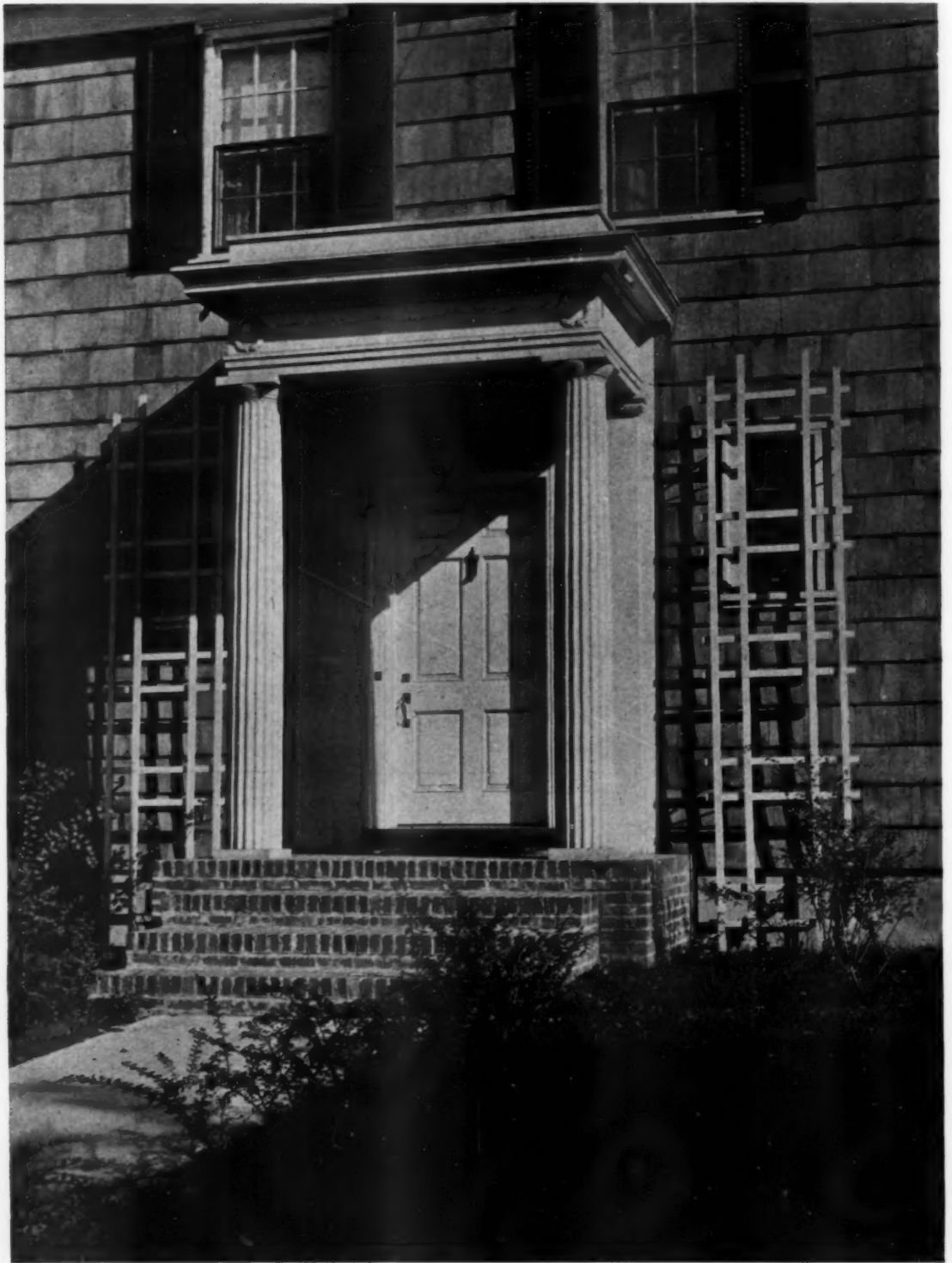
ENTRANCE DETAIL, HOUSE OF G. M. ROSENTHAL, PITTSFIELD, MASS.
