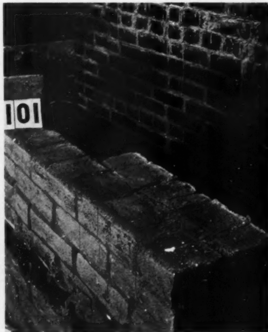
WALL NO. 101 AFTER TEST. BRICKS HAVE BEEN REMOVED TO SHOW TYPICAL BEDDING AS LAID BY MASON B
