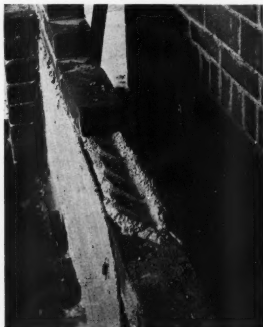
HORIZONTAL MORTAR BED PREPARED BY MASON A. NOTE VERTICAL GROOVING OF MORTAR AND COMPARE WITH WORK OF MASON B
