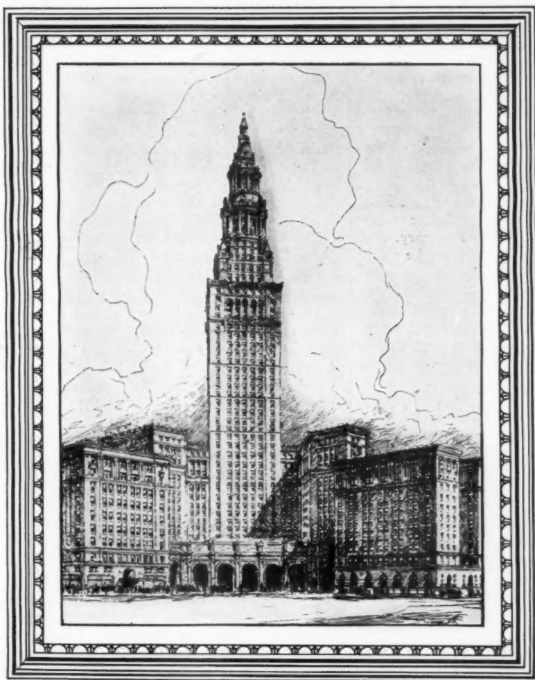
CLEVELAND UNION TERMINAL Cleveland, Ohio
