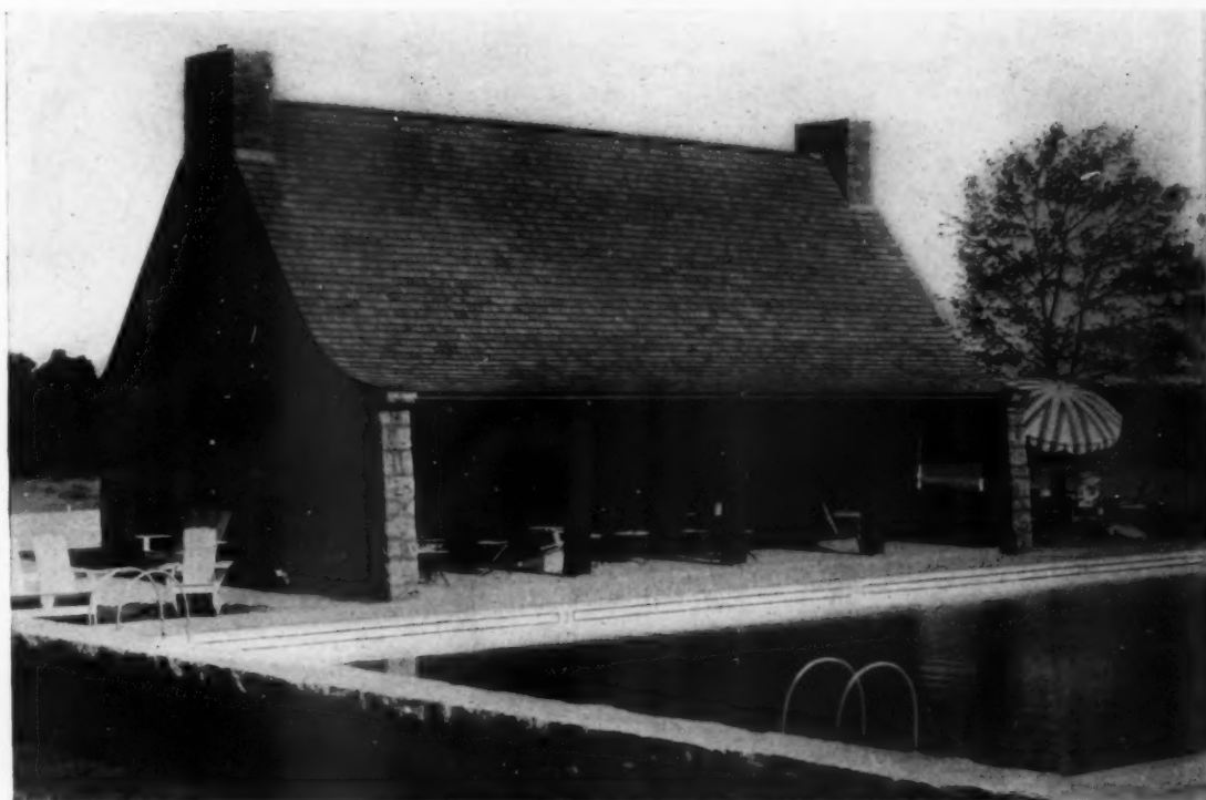
THE LOCKER HOUSE
