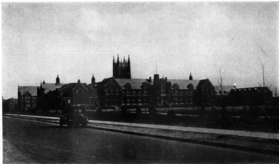
GENERAL VIEW, REAR FACADE
