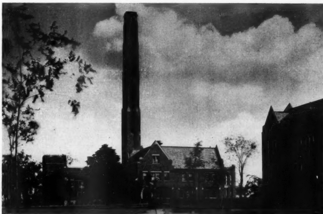
GENERAL VIEW OF THE MECHANICAL PLANT SACRED HEART SEMINARY, DETROIT, MICH. DONALDSON & MEIER, ARCHITECTS
