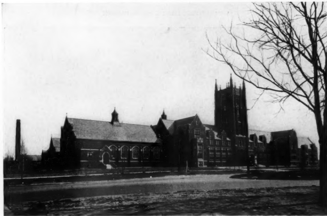
GENERAL VIEW, MAIN FACADE
