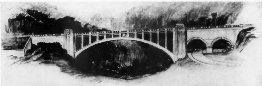
MT. WASHINGTON ROADWAY BRIDGE, PITTSBURGH, PA.
