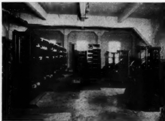
ELEVATOR PENTHOUSE SHOWING ELEVATOR CONTROL APPARATUS
