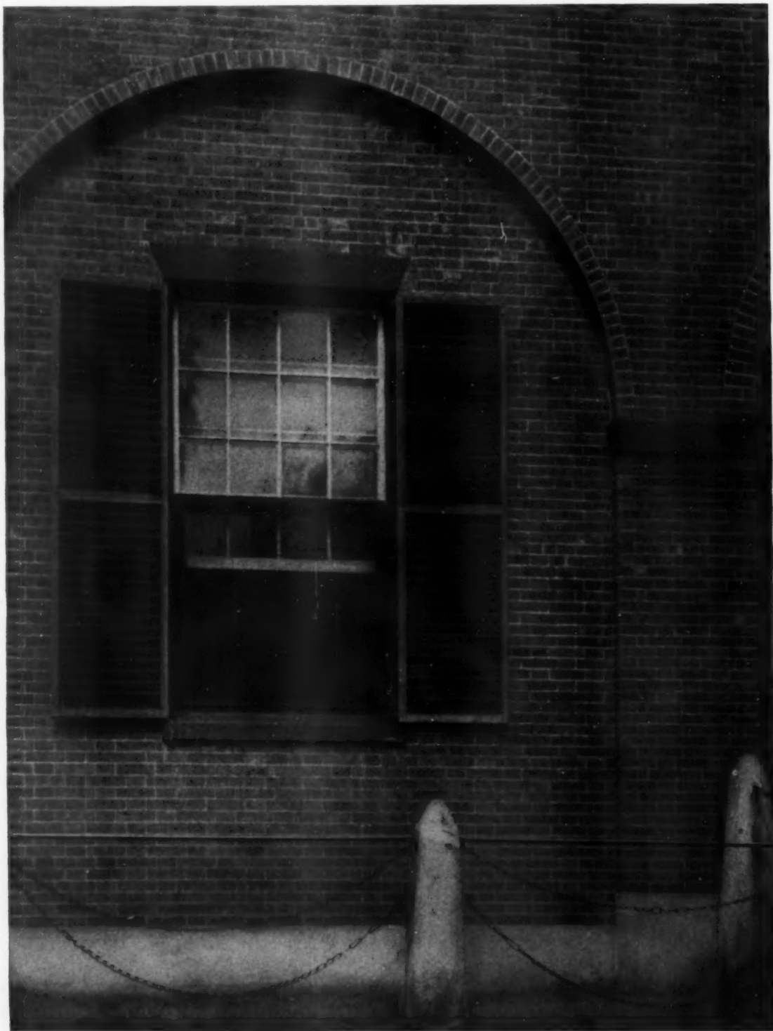
DETAIL OF WINDOW BAY, OLD COURT HOUSE, WISCASSET, ME.
