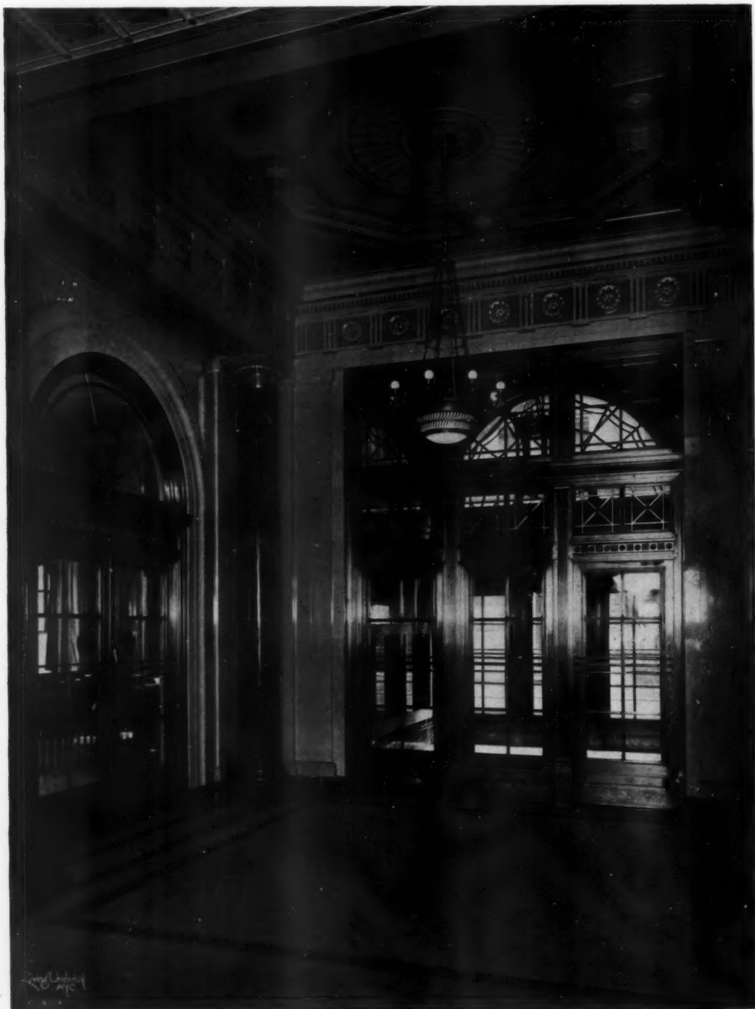
ROYAL BUILDING FOR ROYAL INSURANCE COMPANY, NEW YORK STARRETT & VAN VLECK, ARCHITECTS
