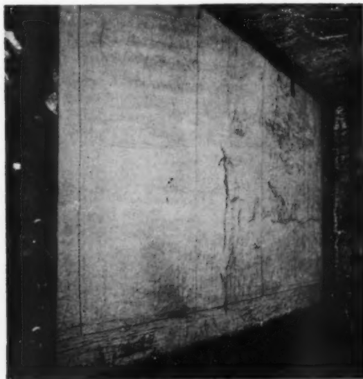
INTERIOR OF TEST HOUSE SHOWING CURTAIN IN PLACE STRETCHED OVER THE STRUCTURAL FRAME, FORMING ONE SIDE OF THE FURNACE AND READY FOR TESTING
