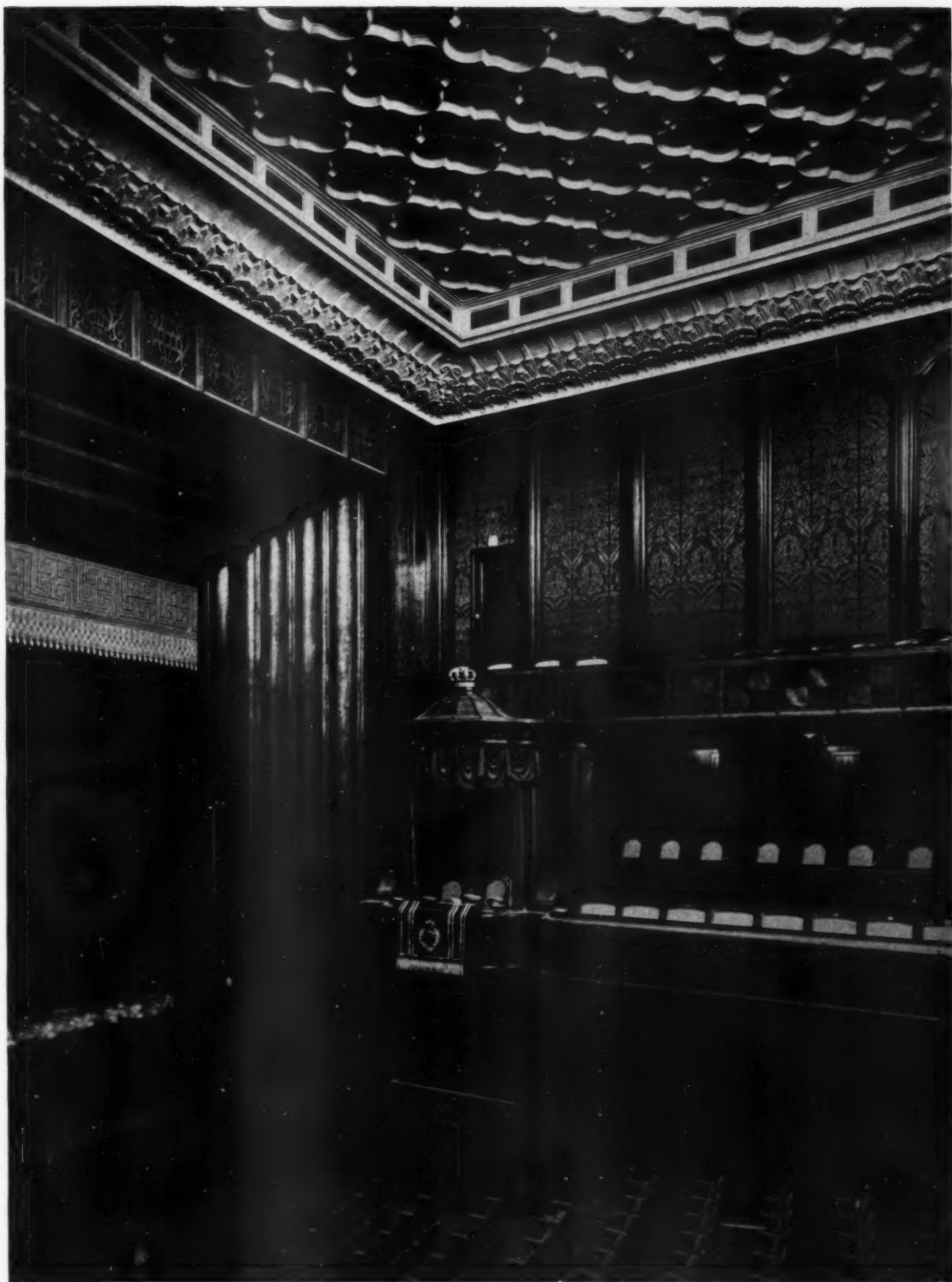
THE PROSCENIUM KLEINES HAUS, LANDESTHEATER, STUTTGART PROFESSOR M. LITTMANN, ARCHITECT
