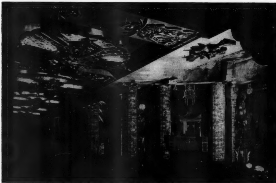
THE AUDITORIUM AND PROSCENIUM
