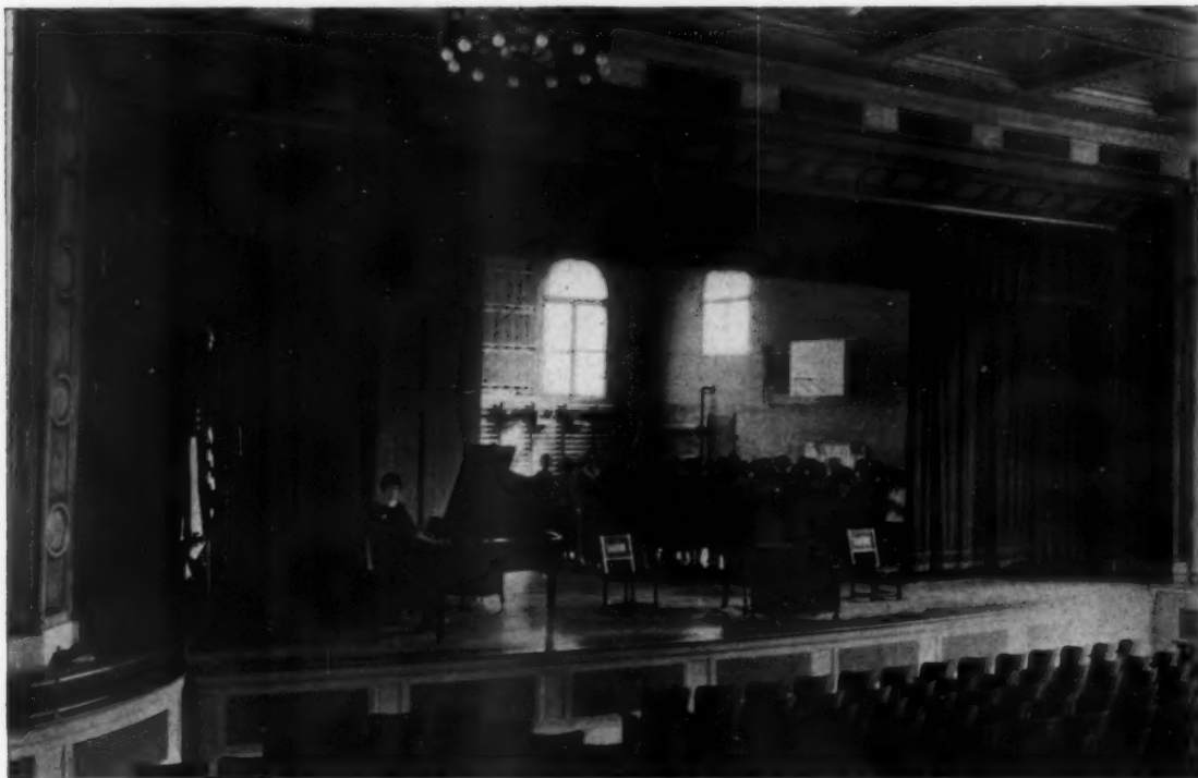
AUDITORIUM, GLASSBORO NORMAL SCHOOL, GLASSBORO, N. J.—GUILBERT & BETELLE, ARCHITECTS
