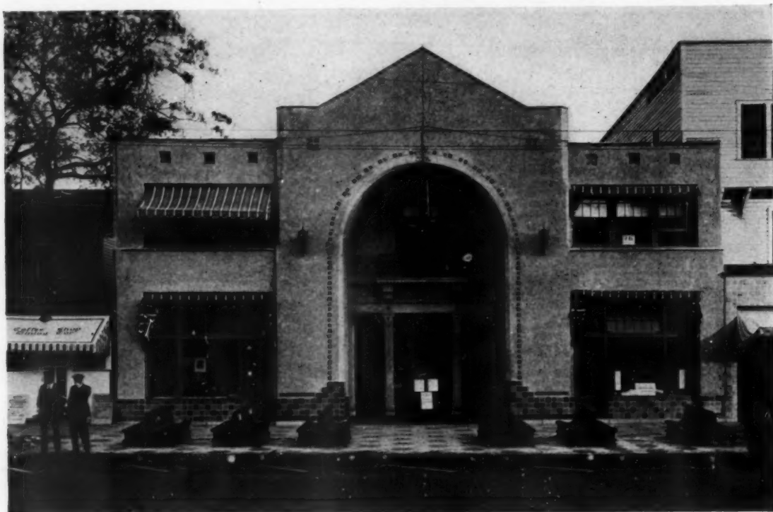
PENN-FLORA ARCADE, ST. PETERSBURG, FLA.—HARRY F. CUNNINGHAM, ARCHITECT
