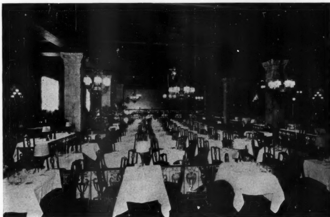
STATLER HOTEL AND OFFICE BUILDING, BOSTON, MASS.
