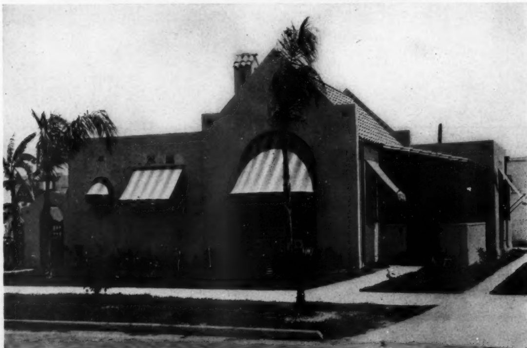
HOUSE OF O. H. BITTING, ST. PETERSBURG, FLA.—HARRY F. CUNNINGHAM, ARCHITECT
