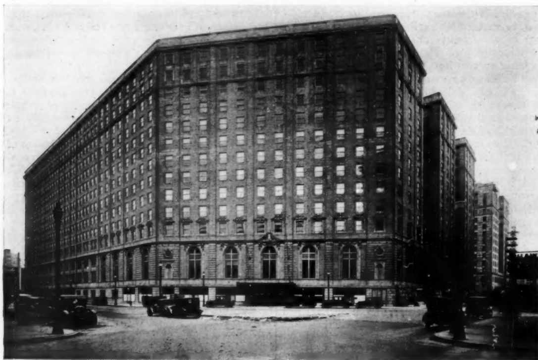
STATLER HOTEL AND OFFICE BUILDING, BOSTON, MASS.
