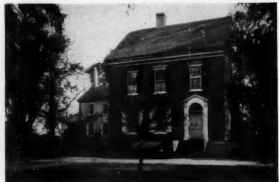
WOODBURN HOUSE, DOVER, DEL.
