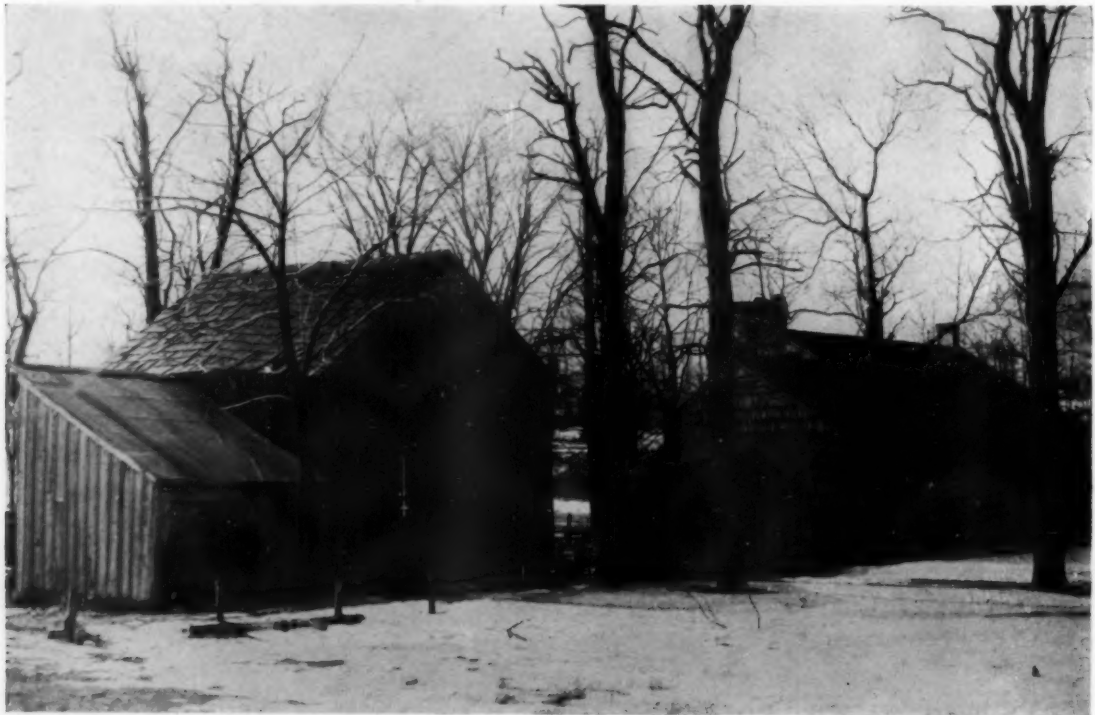
REAR OF OLD HOUSE. SHOWING OLD BARN WHICH WAS REMOVED AT THE TIME ALTERATIONS WERE MADE, AND THE KITCHEN LEANTO AS IT ORIGINALLY APPEARED
