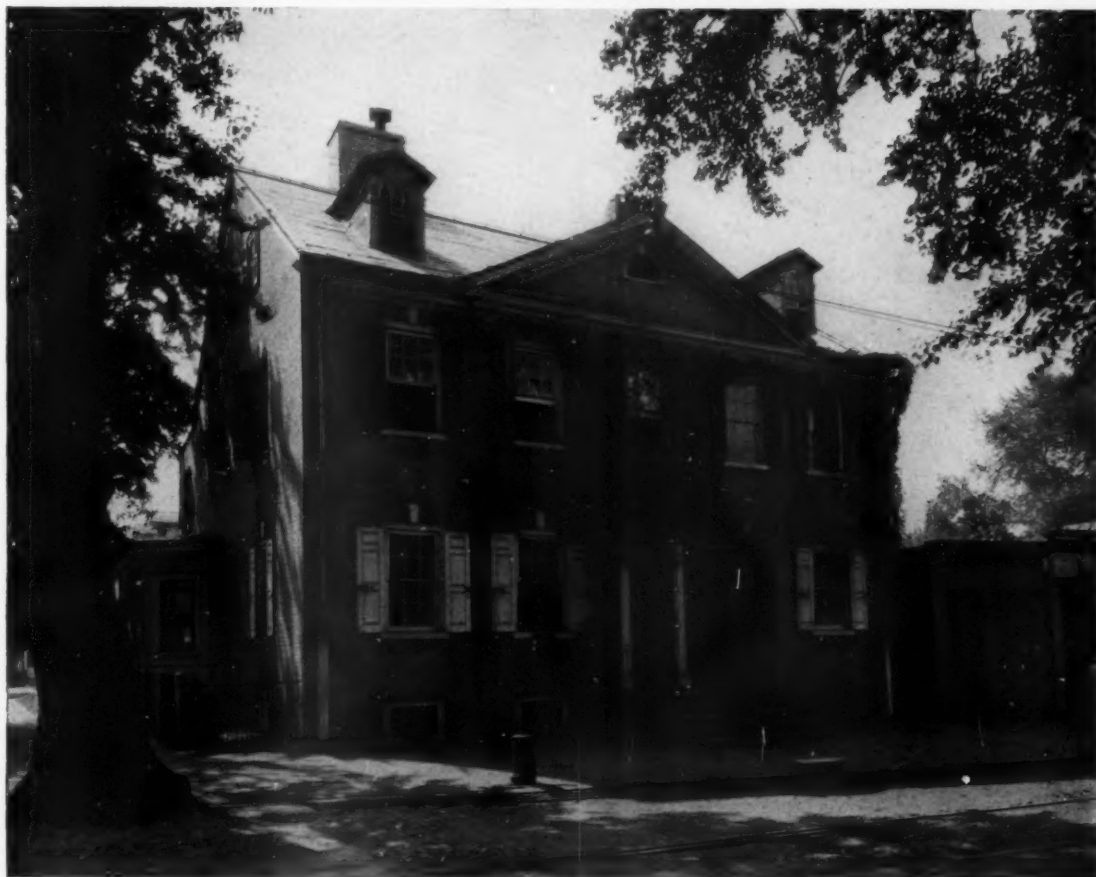
HOUSE ON DELAWARE STREET, NEW CASTLE, DEL.—BUILT 1799
