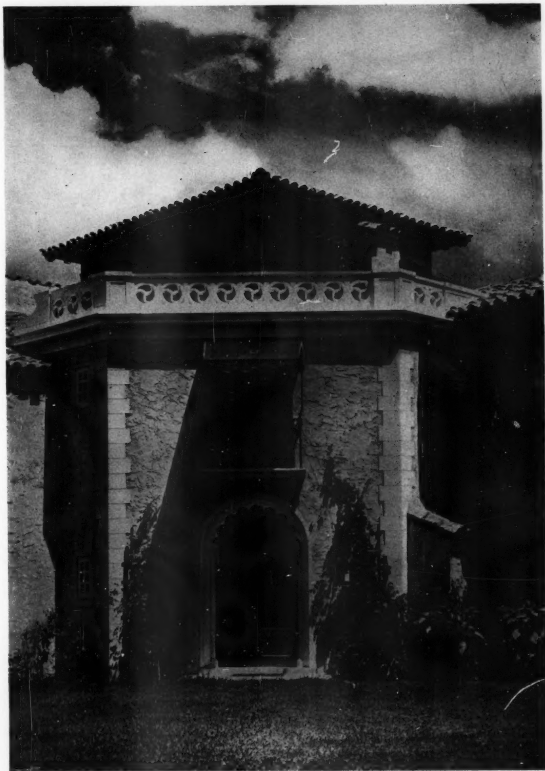
DETAIL OF PRINCIPAL ENTRANCE HOUSE OF GEORGE A. VARNEY, COCONUT GROVE. FLA. WALTER C. DE GARMO, ARCHITECT
