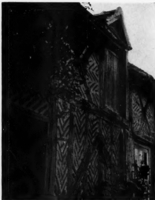
DETAIL OF FARMHOUSE AT COURMEMIN
