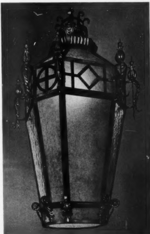
REPRODUCTION OF A PHOTOGRAPH OF AN INTERESTING LANTERN WITH BULB LIGHTED. THE SOURCE OF LIGHT IS PLACED AT THE LINE OF BUOYANCY, THEREBY INCREASING ITS EFFECTIVENESS BOTH AS A DECORATIVE FIXTURE AND AS A UNIT OF THE SYSTEM OF ARTIFICIAL LIGHTING
