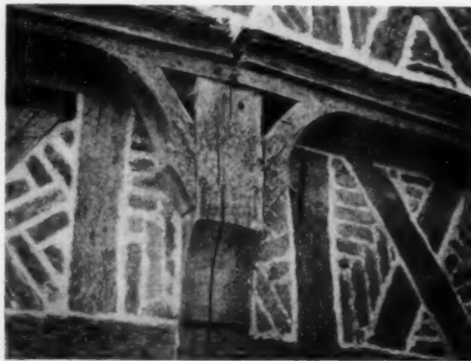
DETAIL OF SUPPORTING BRACKET, HOUSE AT COURMEMIN
