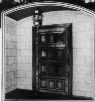
Main Entrance Door. Solid oak, 4' x 8', 3" thick with boiler plate inserted in middle of door. Total weight 700 lbs. Mounted on 4 extra heavy Stanley Ball Bearing Butts.
