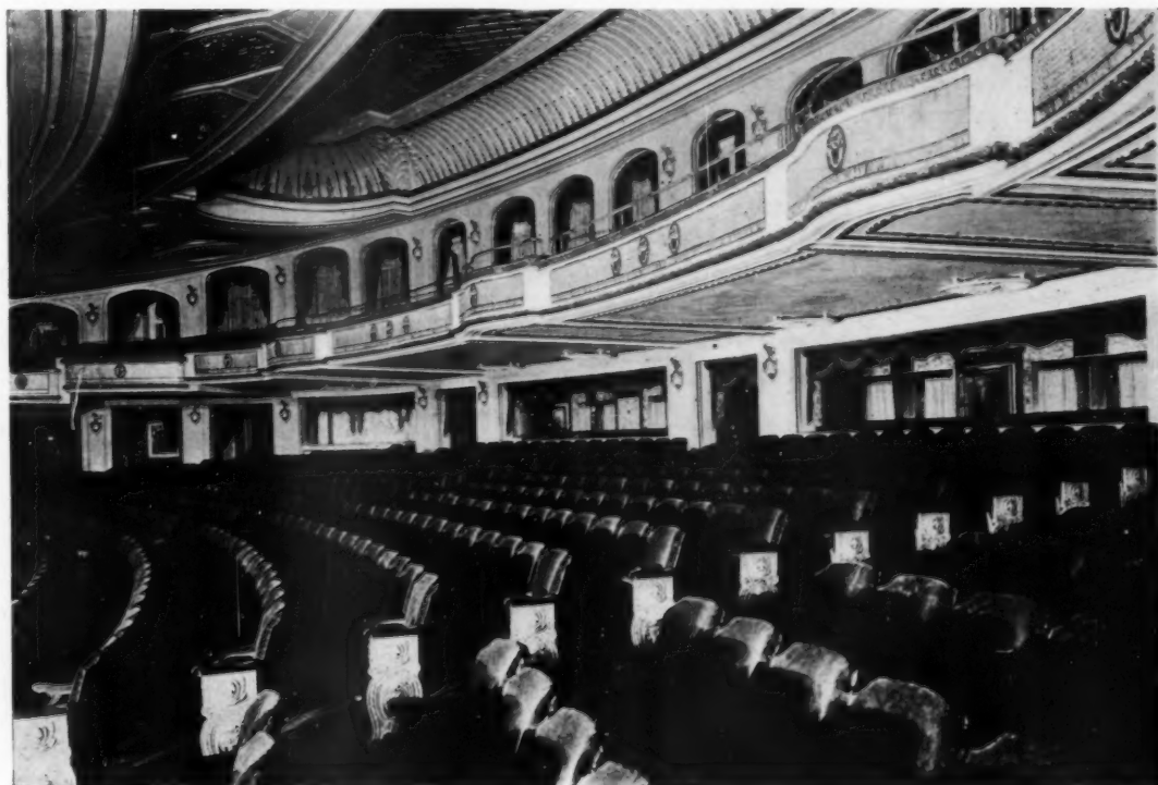
GENERAL VIEW OF LOGES AND BALCONY SOFFIT
