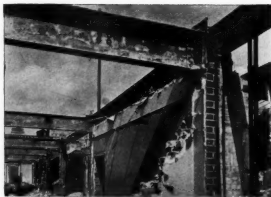
BLENHEIM APARTMENTS, PHILADELPHIA, ERECTED IN 1901, DEMOLISHED IN 1927. STEELWORK AS CLEAN AND IN AS GOOD CONDITION AS WHEN FIRST ERECTED
