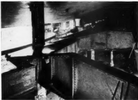
FORREST THEATRE, PHILADELPHIA, ERECTED IN 1905. DEMOLISHED IN 1927. BALCONY GIRDERS AND STEELWORK CLEAN AND FREE FROM CORROSION
