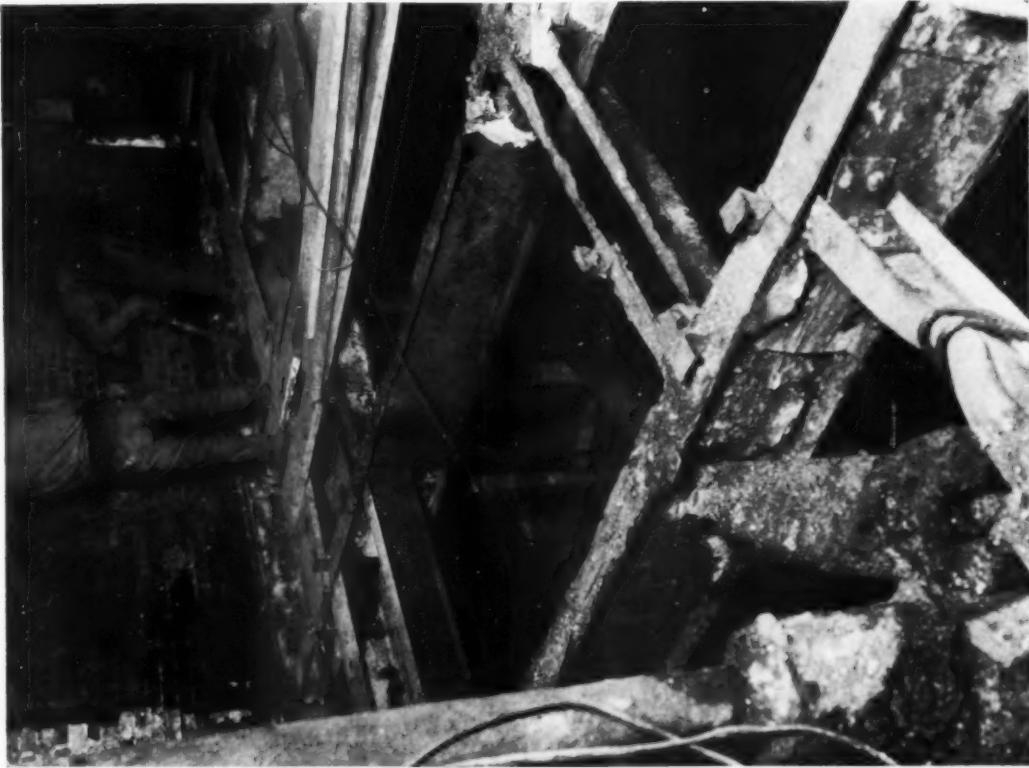
BOILER AND COAL ROOM WHERE WATER RAN OVER SLACK ILLINOIS BITUMINOUS COAL. DISSOLVED ACIDS PENETRATED THE FIREPROOFING AND DESTROYED THE PROTECTIVE PAINT ON THE STEELWORK, CAUSING CORROSION OF THE STEELWORK. UNDER THESE CONDITIONS STEEL MUST BE PROTECTED WITH AN ACID-PROOF COATING, AND THE FIREPROOFING EITHER OF TILE OR CONCRETE MUST BE ABSOLUTELY WATERPROOF AND ACID-RESISTING. NO CORROSION FOUND IN OTHER PARTS OF THE STRUCTURE
