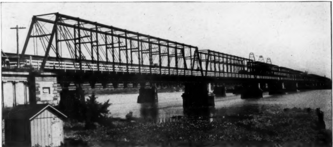
SUSQUEHANNA RIVER BRIDGE AT HAVRE DE GRACE, MD. OPENED FOR RAILROAD TRAFFIC IN 1878 BY THE PENNSYLVANIA RAILROAD COMPANY. CONVERTED TO A HIGHWAY TOLL BRIDGE IN 1910. AN UPPER DECK ROADWAY INSTALLED FOR TWO-WAY TRAFFIC IN 1927. ORIGINAL METAL IN PERFECT CONDITION
