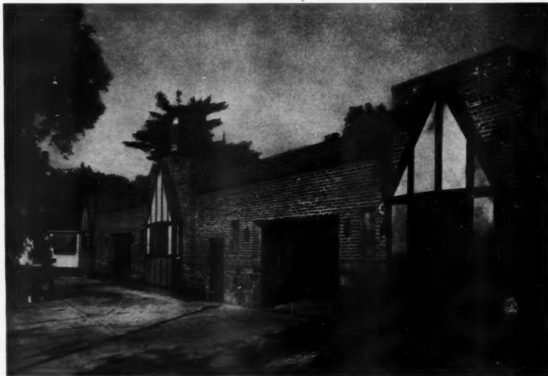
PRIVATE GARAGE, BLIND BROOK LODGE APARTMENTS, RYE, N. Y. VAN WART & WEIN, ARCHITECTS
