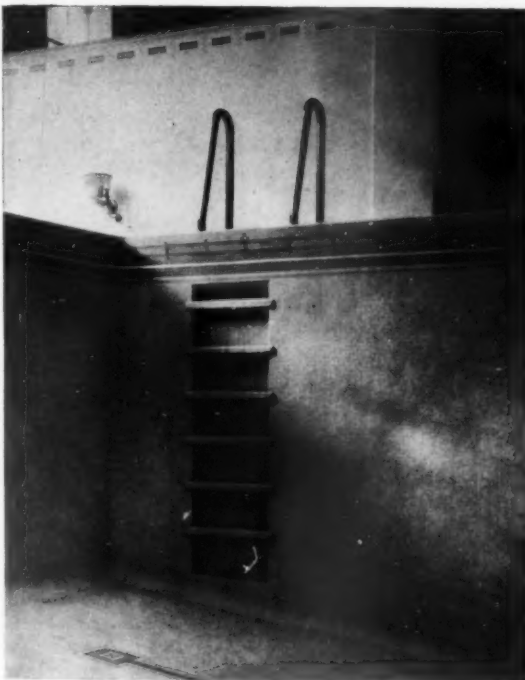
LIBERTY HIGH SCHOOL, BETHLEHEM, PA. VERUS T. RITTER, ARCHITECT
