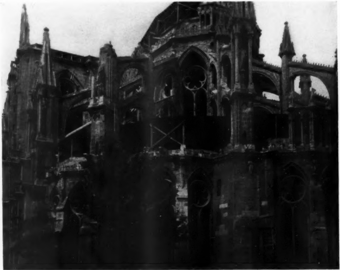
RHEIMS CATHEDRAL—CONSTRUCTION OF THE APSE
