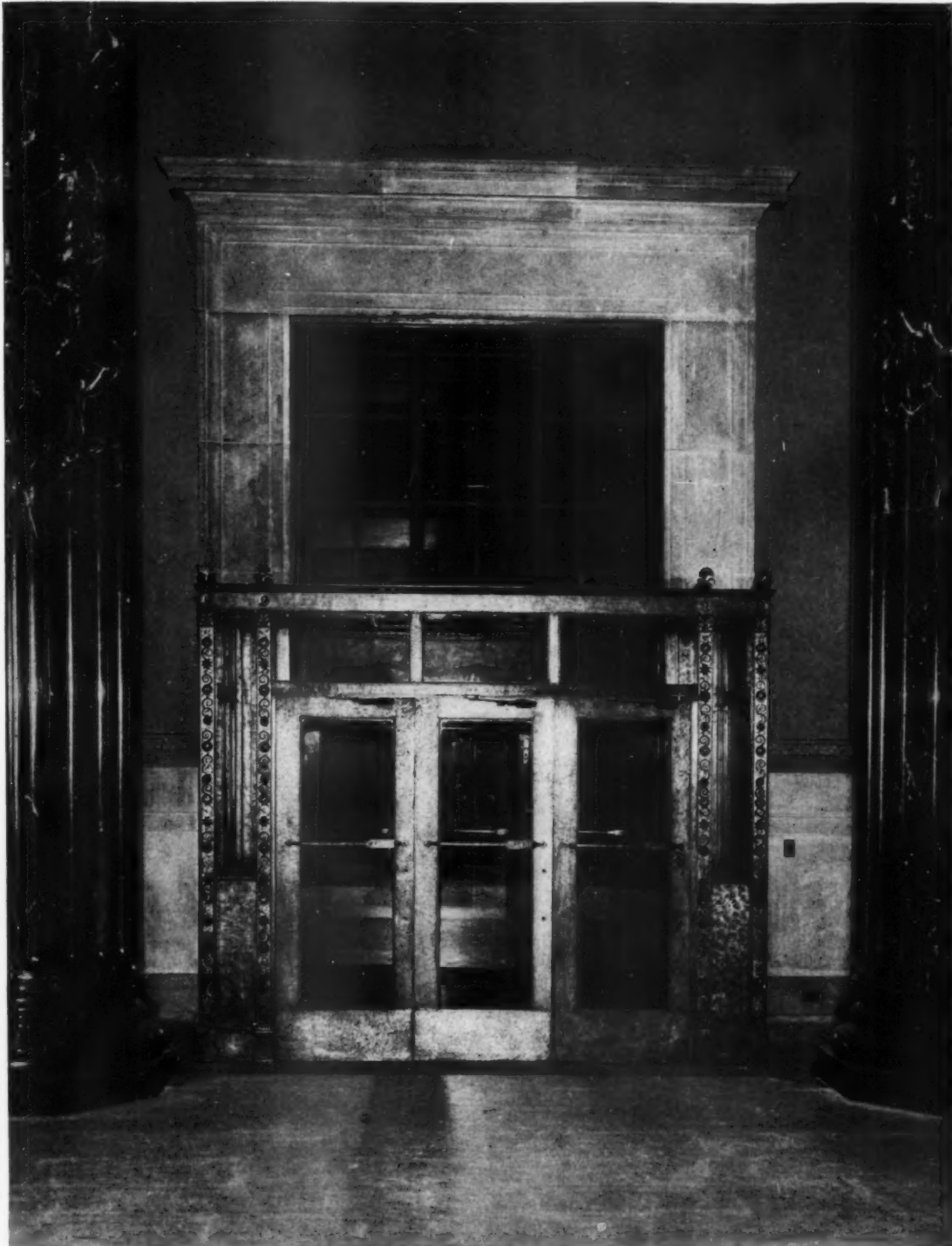
THE ENTRANCE IS OF WROUGHT IRON IN INTERESTING DESIGN. THE CASING OF THE DOOR OPENING IS OF INDIANA LIMESTONE. THE WALLS OF THE BANKING SPACE ARE OF INDIANA LIMESTONE WITH A MIXTURE OF ABOUT TEN PER CENT OF BRIAR HILL STONE
