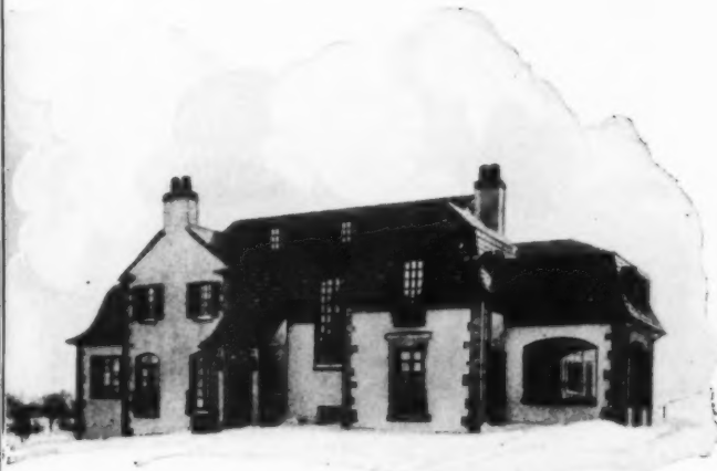
Residence of E. W. Christ, New Britain, Conn. Architects, Perry & Bishop, New Britain, Conn. Stanley Ball Bearing Butts used throughout
