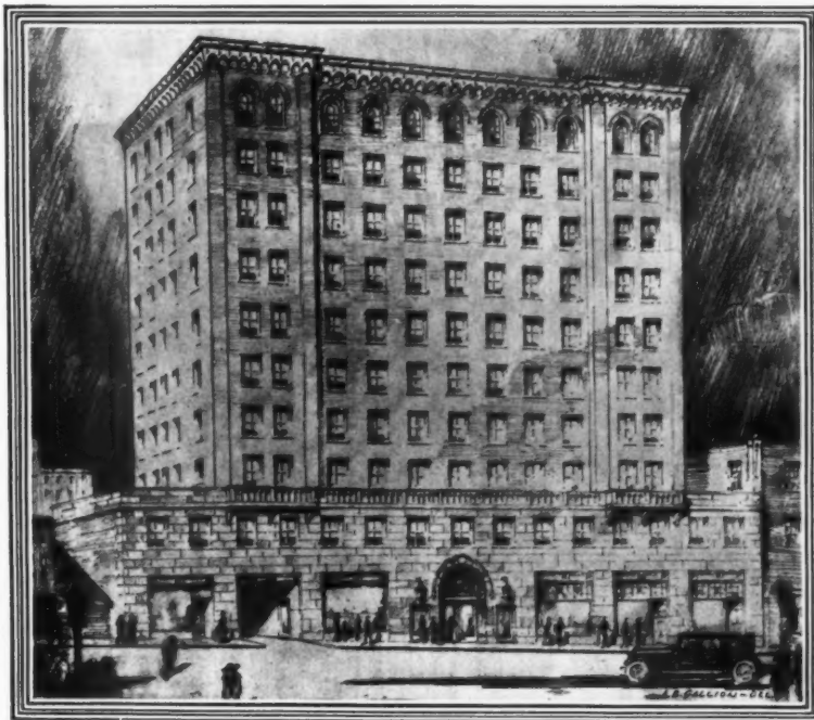
BEAUMONT MEDICAL OFFICE BUILDING St. Louis, Missouri
