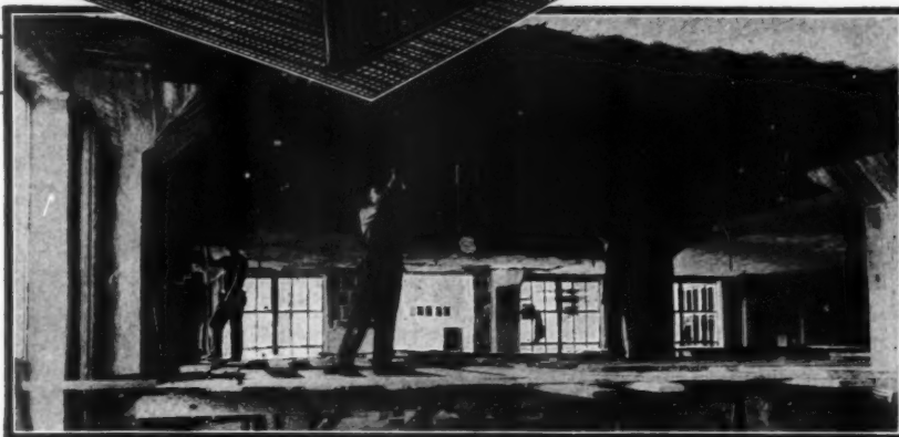
Below: Lathers erecting suspended ceiling of Milcor Netmesh Metal Lath, Journal Building, Milwaukee. Plasterers following up immediately. Notice portion of plastered ceiling.
